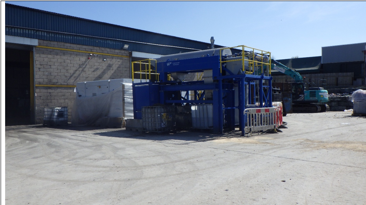
ZX separation technology unit, roller shutter doors in open position.
