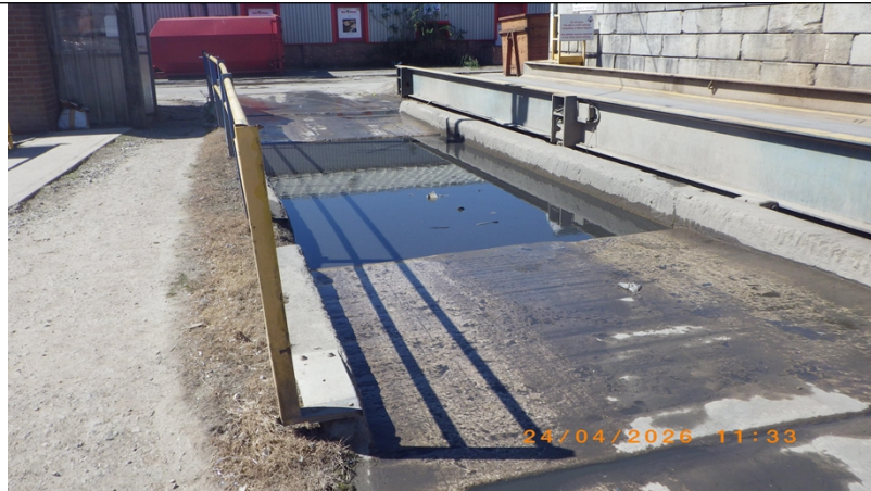
Dust suppression measures observed on site
