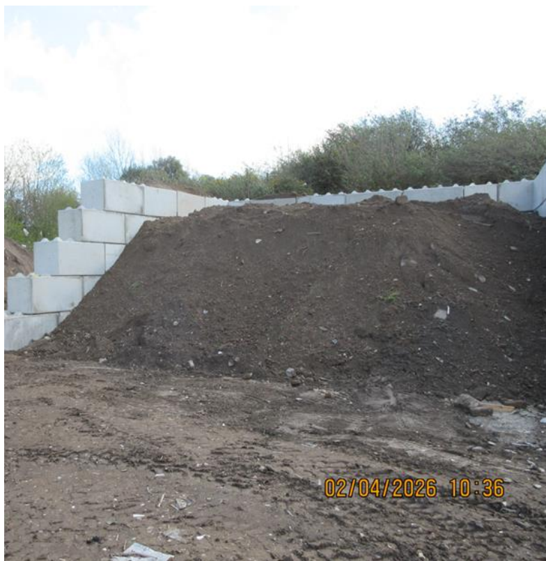
Photograph 6- 1 metre freeboard space at the top of the trommel fines stockpile.
