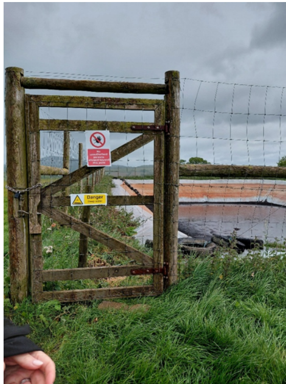
Image 1: Locked gate and fence to the lagoon.
