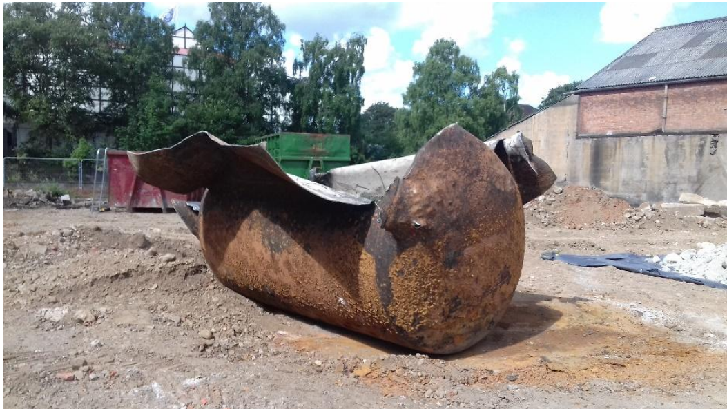
Figure 1. Steel tank inspected on the surface after tank pull.
