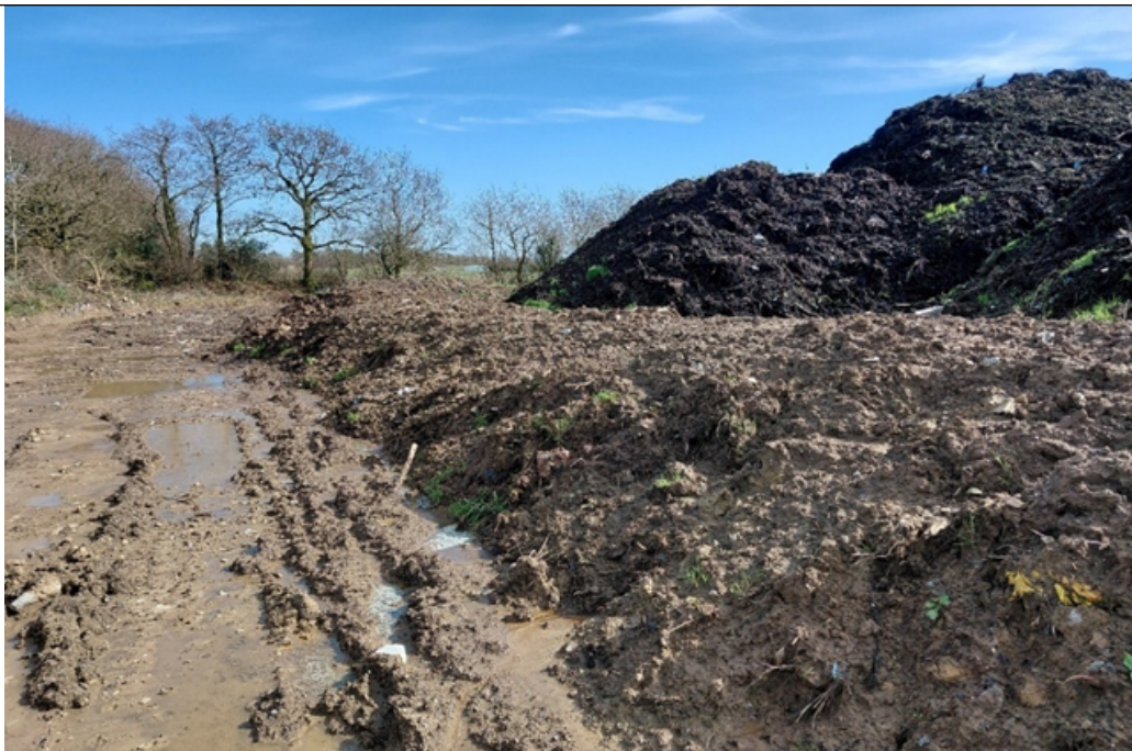
Figure 17 Photo showing additional clay bunding installed to base of old green waste stockpile.
