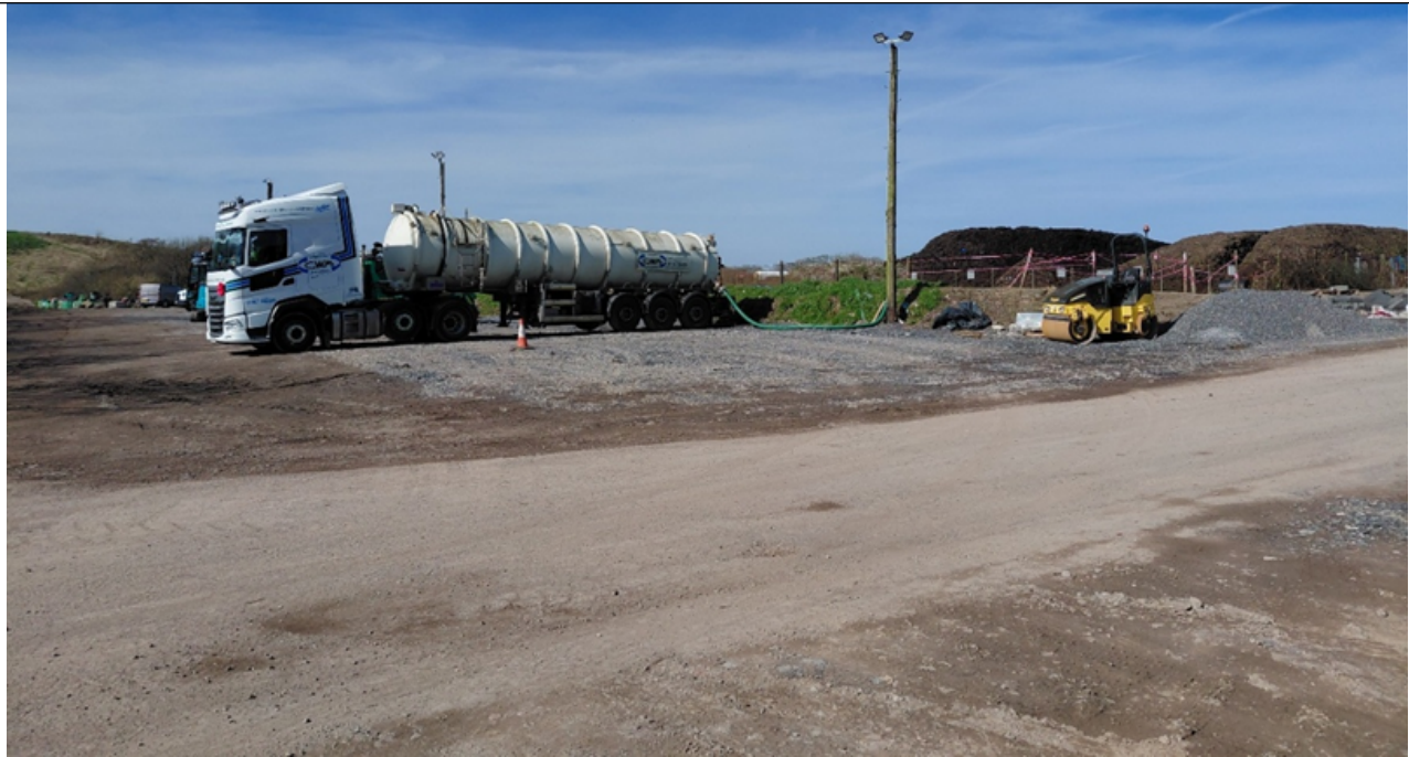
Figure 21 Photo showing leachate removal to tanker at southern side of leachate lagoon.
