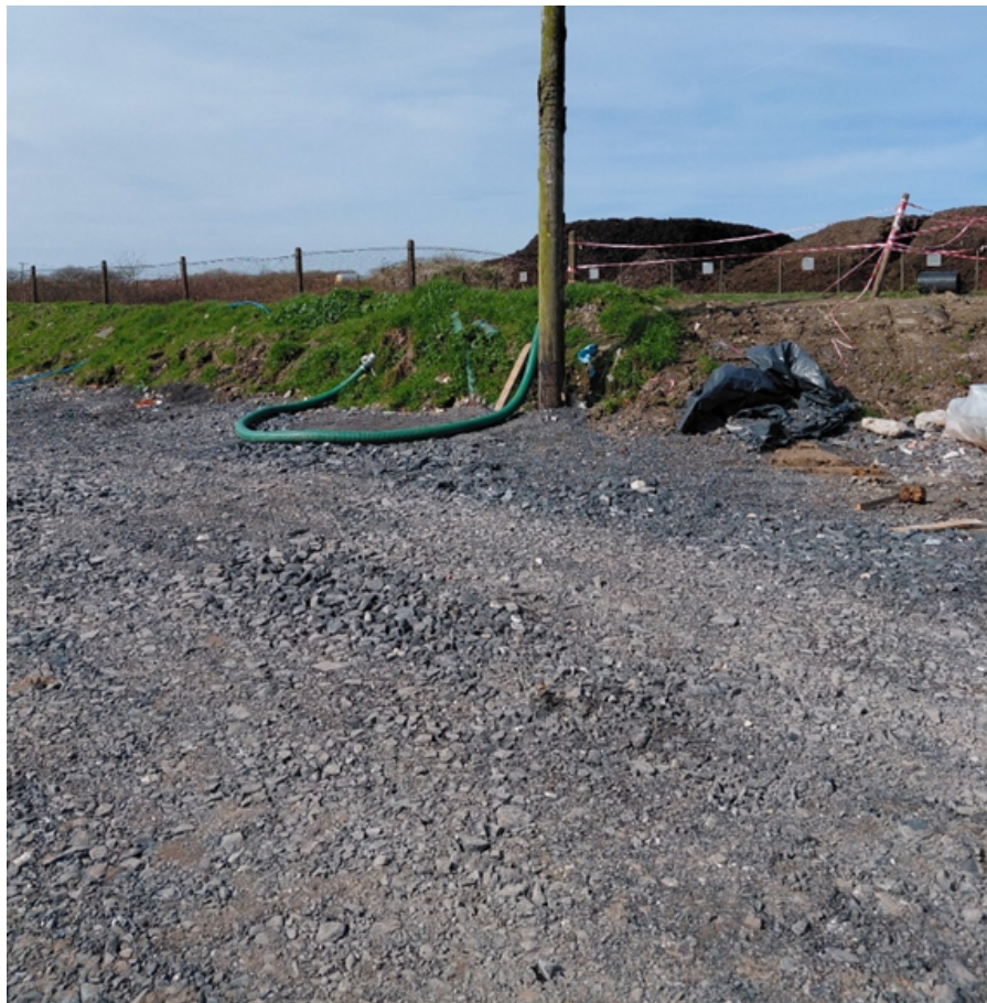
Figure 20 Photo showing southern location leachate removal being taking from.
