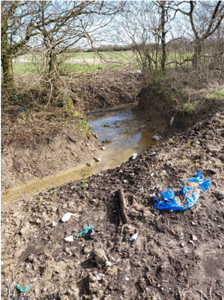
Figure 16 Photo showing newly dug drainage ditch to north of compost pad.
