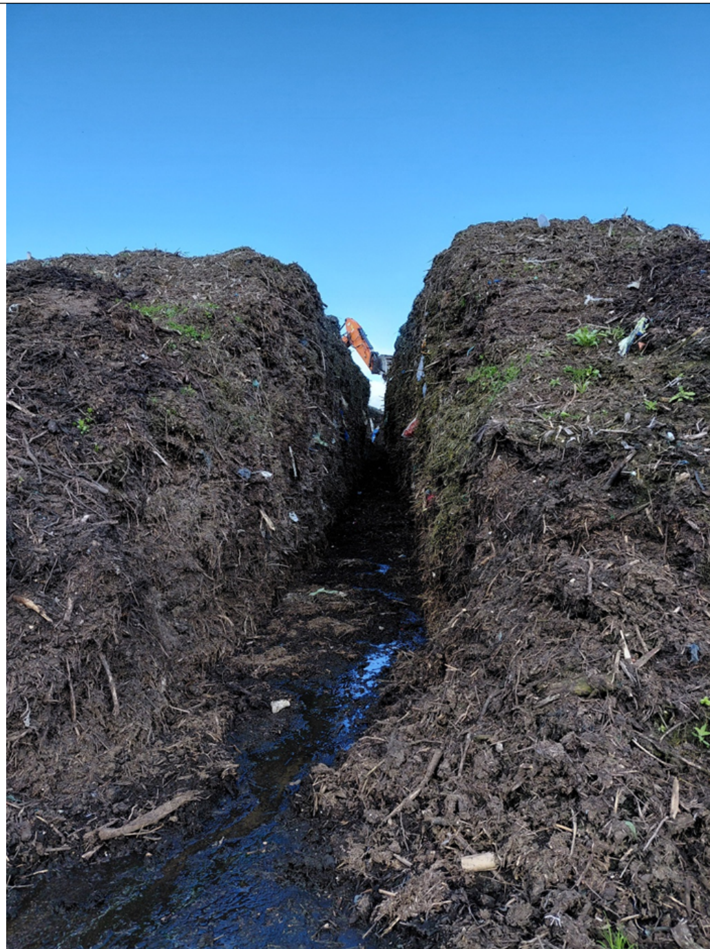
Figure 2 Further photo of legacy green waste stock pile with poorly formed fire break
