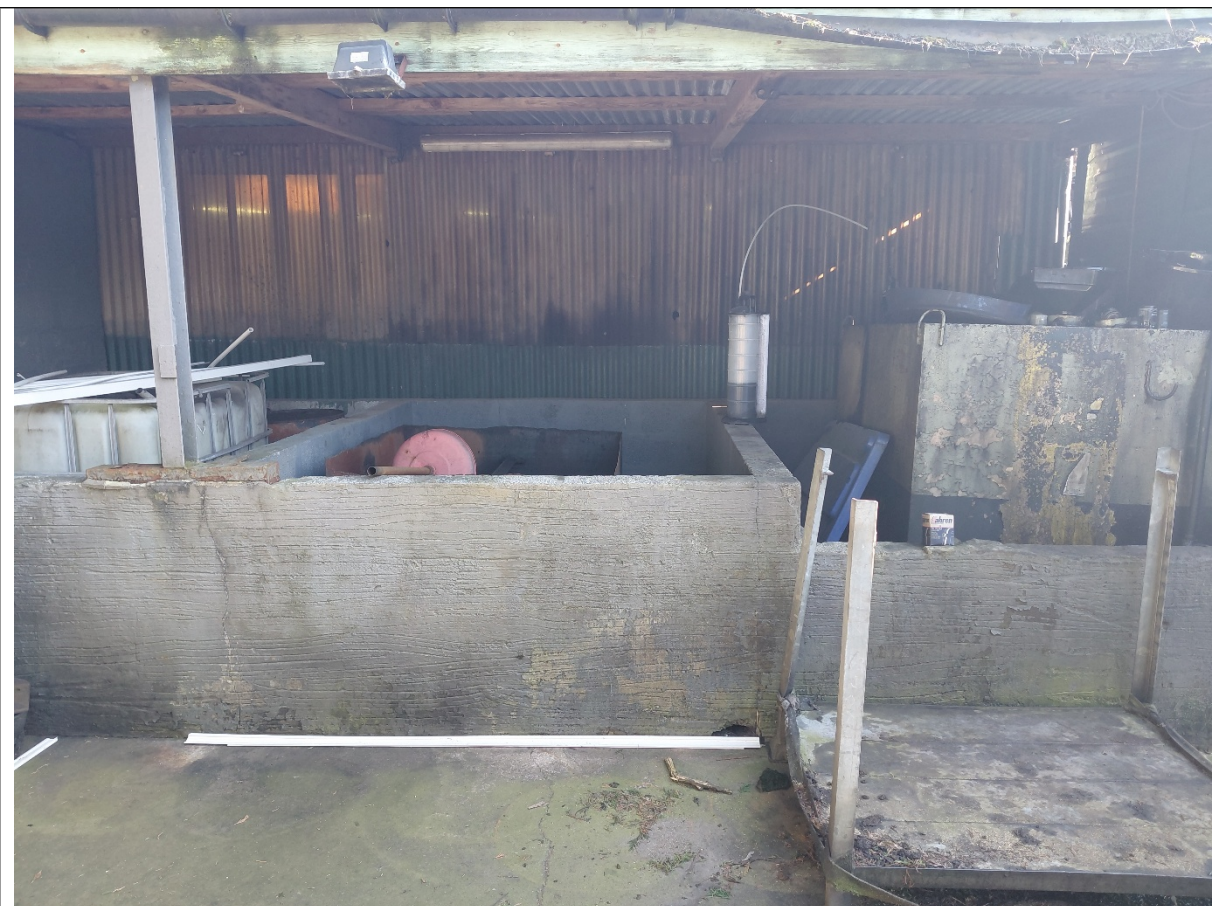
Photograph 3 – waste oil storage within bund wall
