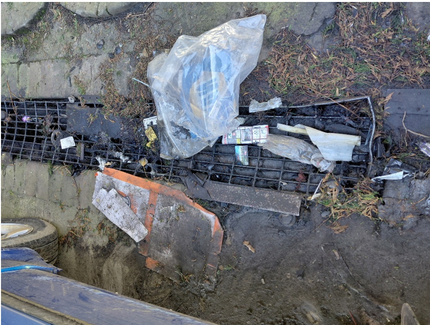
Photograph 1- A photo of the interceptor drain
