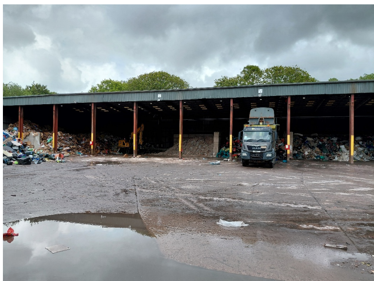
Photo 2 – Waste sorting shed, complete with heat detectors
