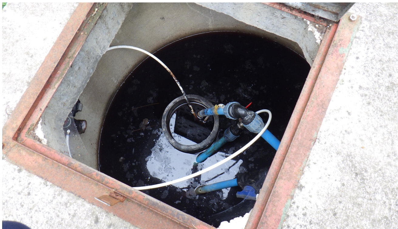
Photograph showing inside of sump 5
