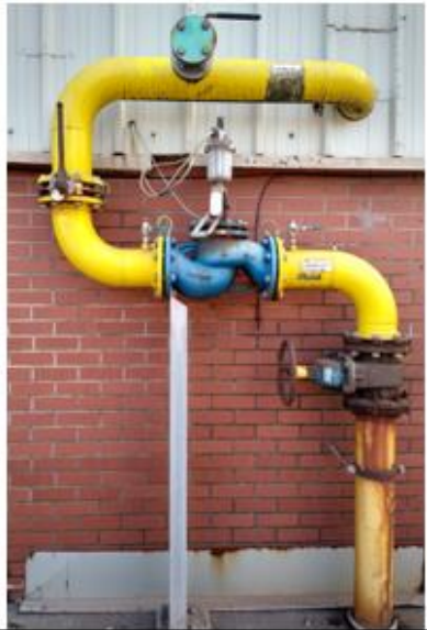
Natural Gas Manual Safety Shut Off Valve
