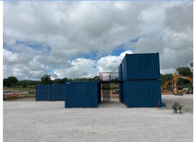
Photograph 4: New welfare and compacted MOT
