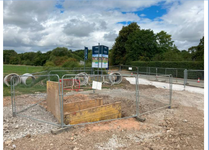
Photograph 8: Trench support in drainage area
