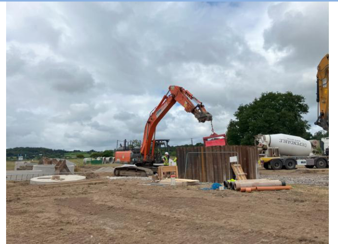
Photograph 8: Drain installation in southern road area
