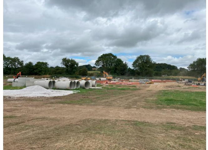
Photograph 2: Storage area in central site area
