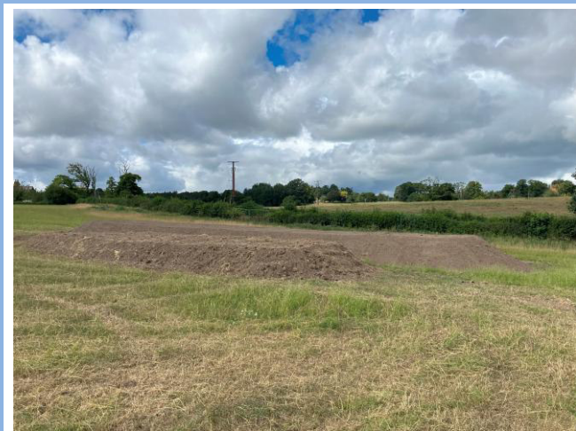
Photograph 9: TS and sod stockpiles
