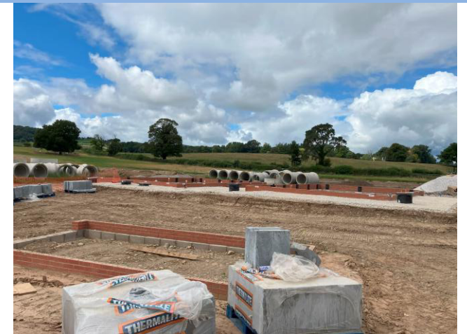
Photograph 6: Foundation bases in northern end of site
