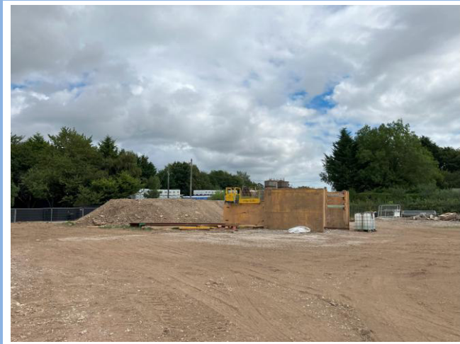
Photograph 7: Trench support and stockpile near vehicle entrance
