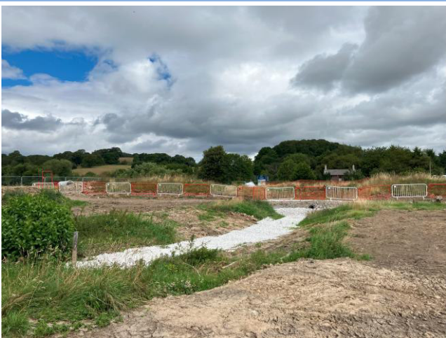
Photograph 3: Historical sluice with drainage gravel
