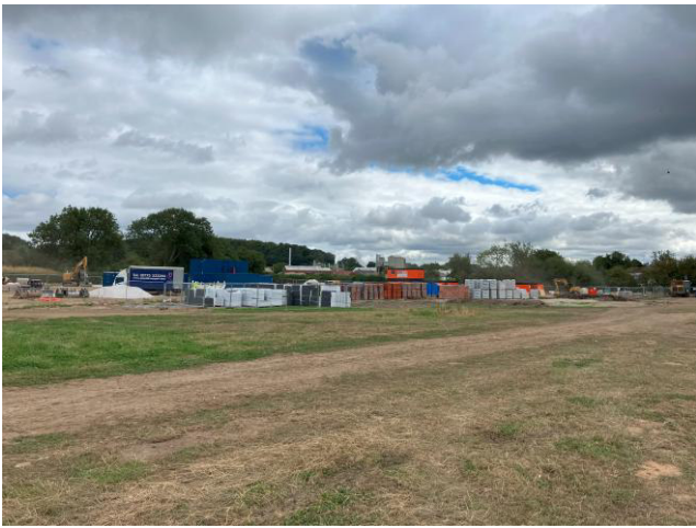
Photograph 1: Storage area in central site area
