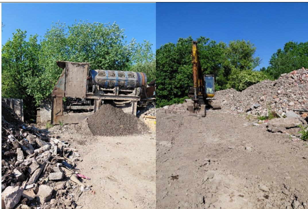
Images 3 and 4: Left – Photograph of the trommel at the rear of site. Right – Photograph of processed hardcore stored at the top of the site.
