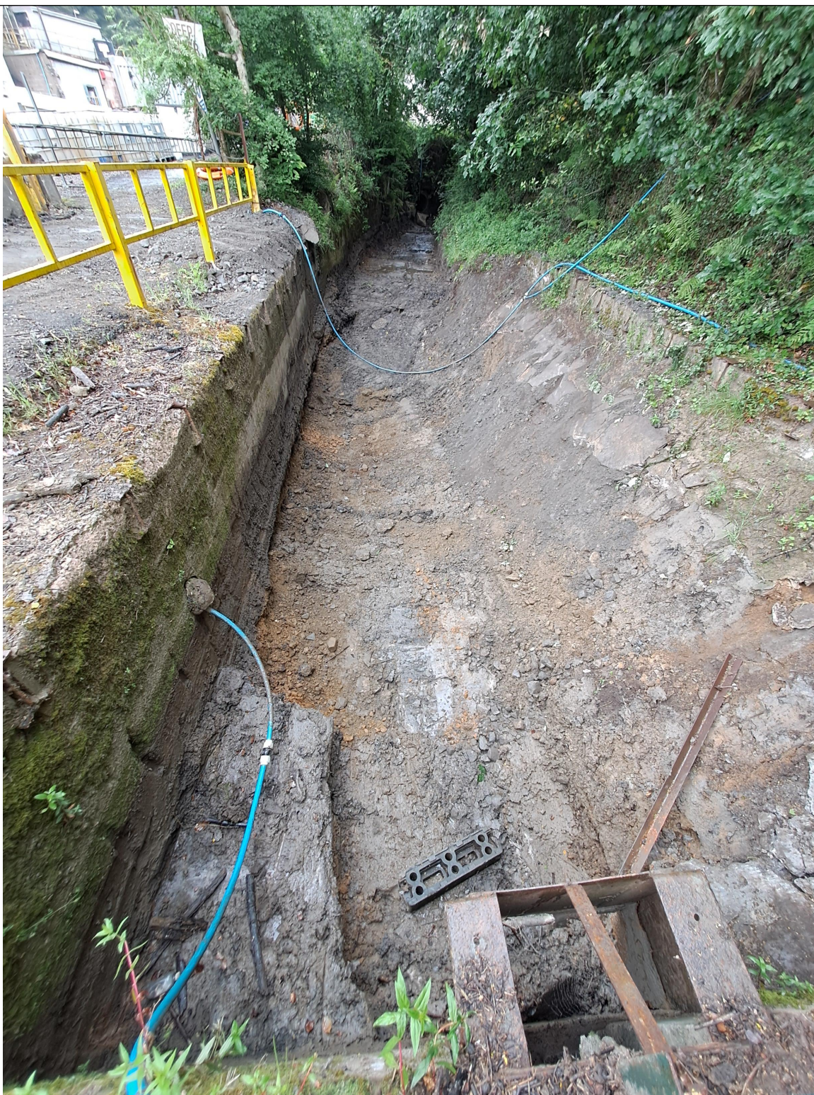
Figure 2 – The final settlement tank as observed during the visit.
