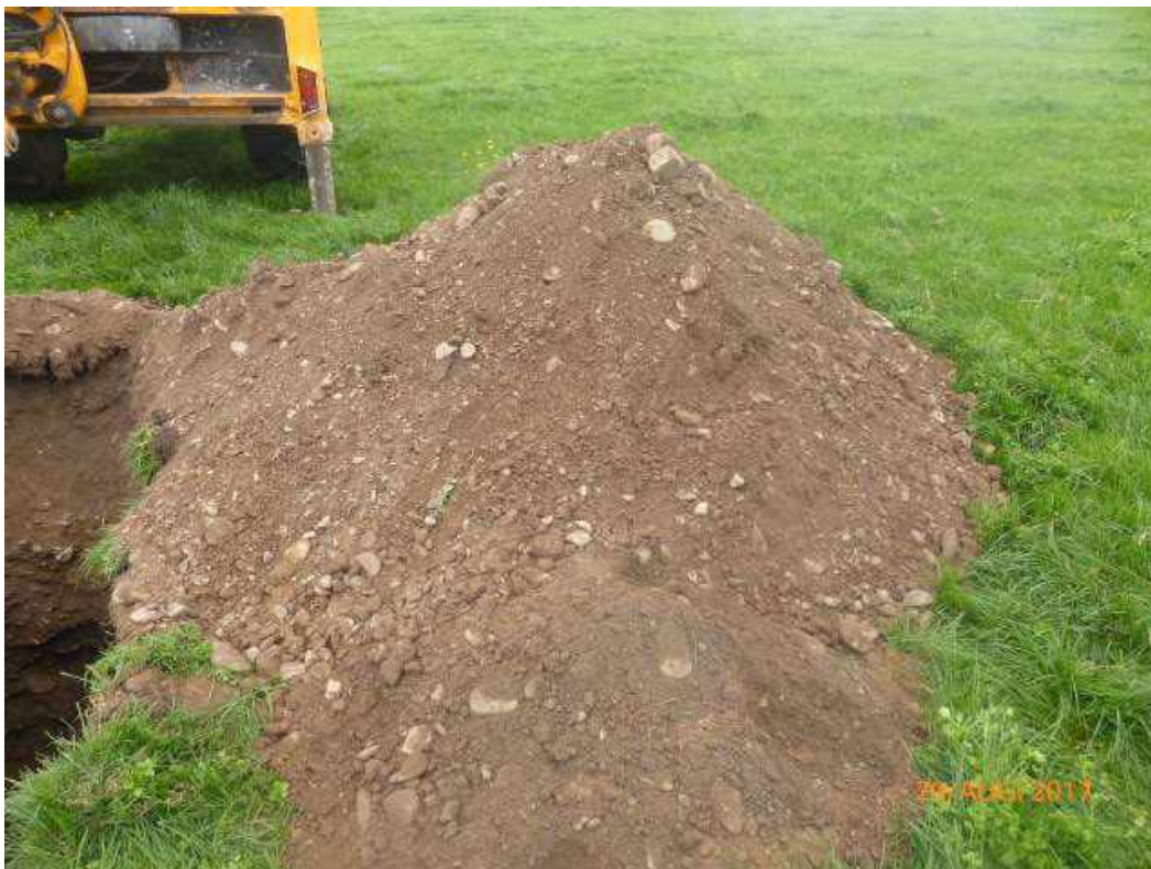
Photo 16 – Arising's from Trial Pit 08
