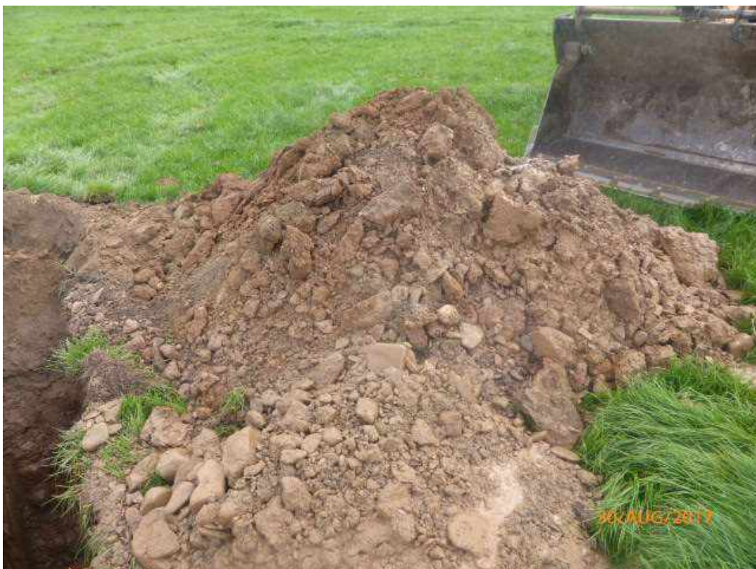
Photo 44 – Arising's from Trial Pit 22
