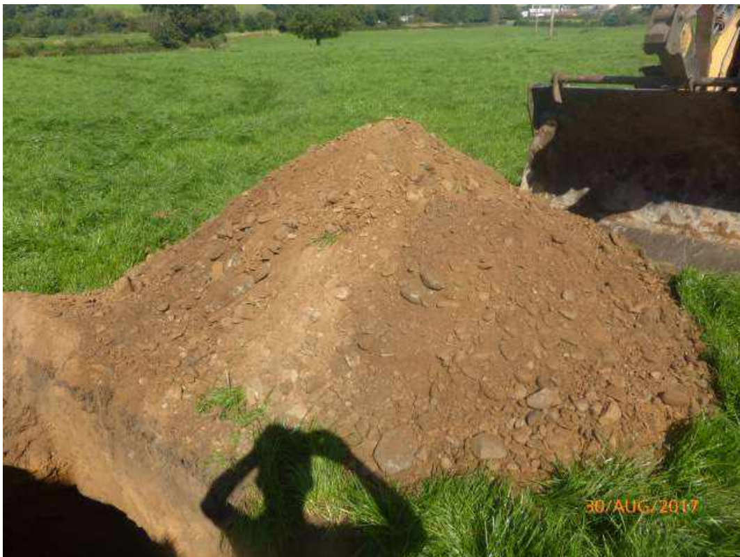
Photo 58 – Arising's from Trial Pit 29
