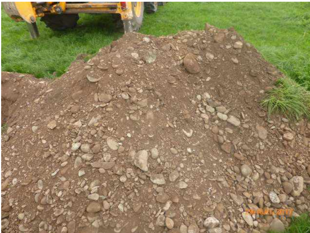
Photo 46 – Arising's from Trial Pit 23
