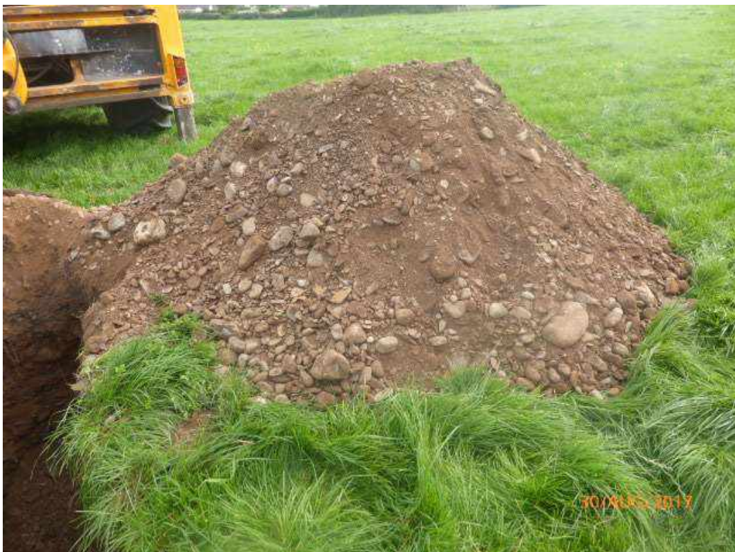
Photo 30 – Arising's from Trial Pit 15
