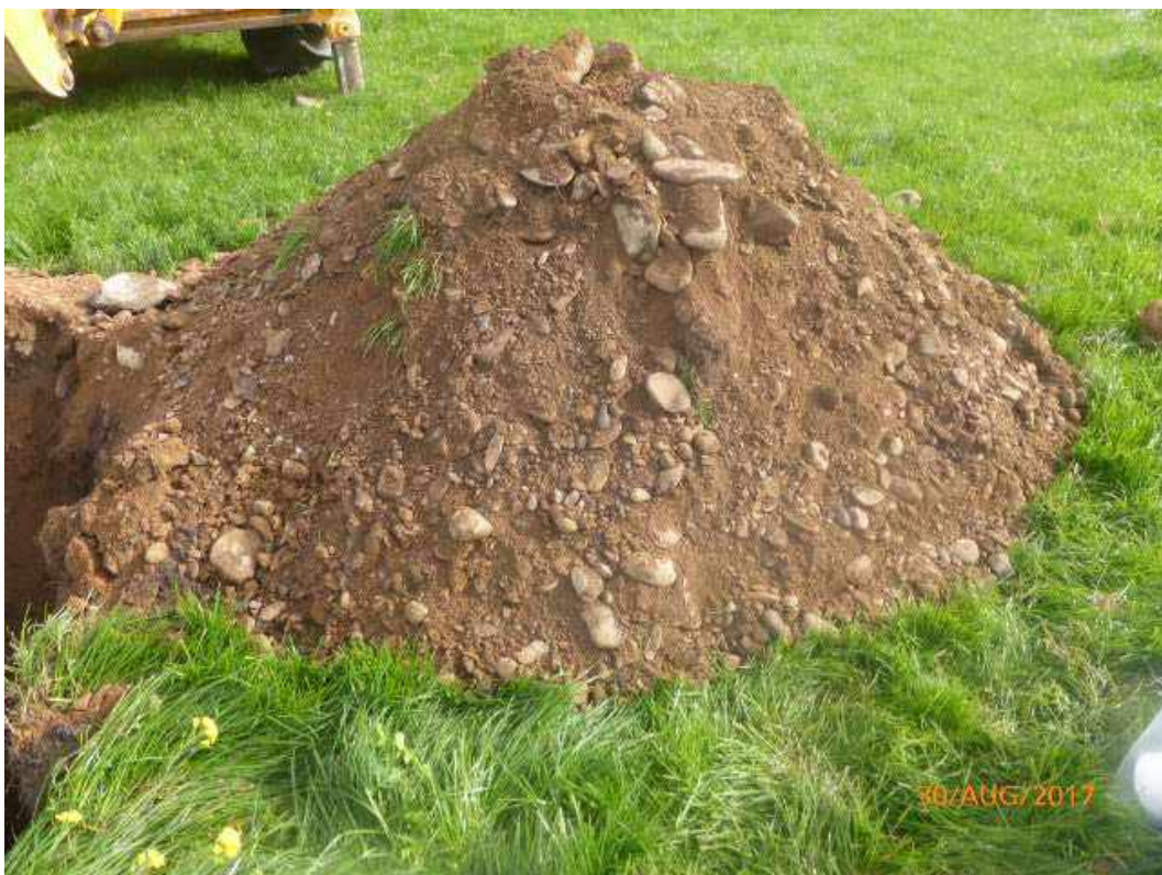
Photo 56 – Arising's from Trial Pit 28
