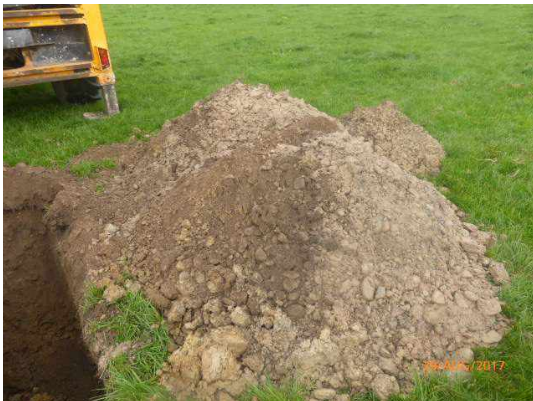
Photo 8 – Arising's from Trial Pit 04
