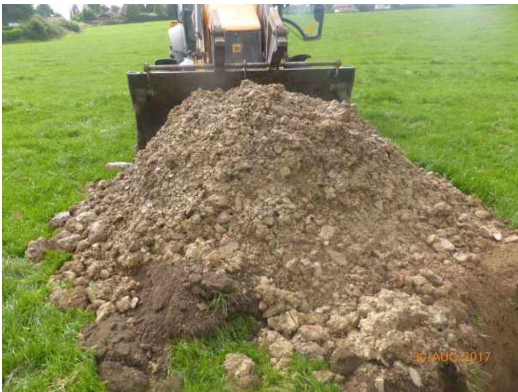
Photo 48 – Arising's from Trial Pit 24
