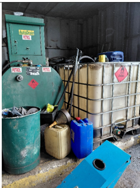
Image 4: Liquids from ELV depollution activities in labelled containers with no direct secondary containment.
