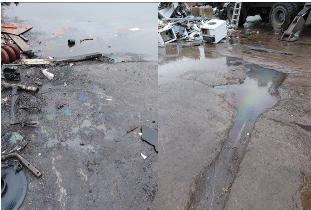
Images 5 and 6: Left – Oil next to a non-depolluted engine. Right – Oil in the drainage channel connected to the sealed sump.
