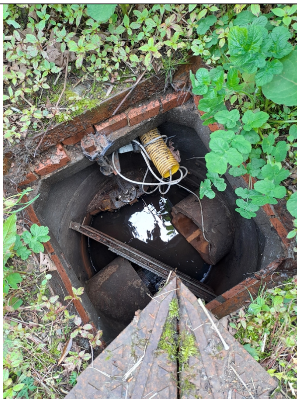
Figure 2 – Chamber lifted where site drainage was observed entering but not leaving during the visit.
