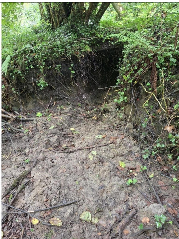
Figure 1 – The conditions of the sample/discharge point similar to that observed during the visit.
