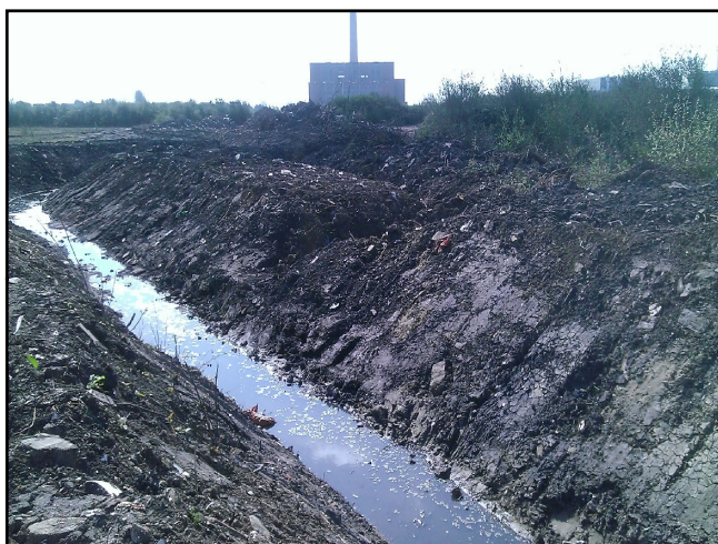
Photograph 6: TN2 - Recent drainage works at the south west of the site.
