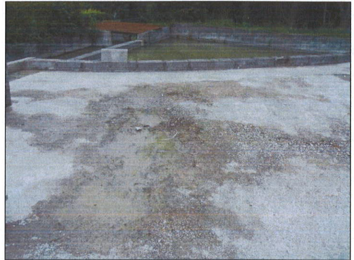
Concrete dust residue in site corner
