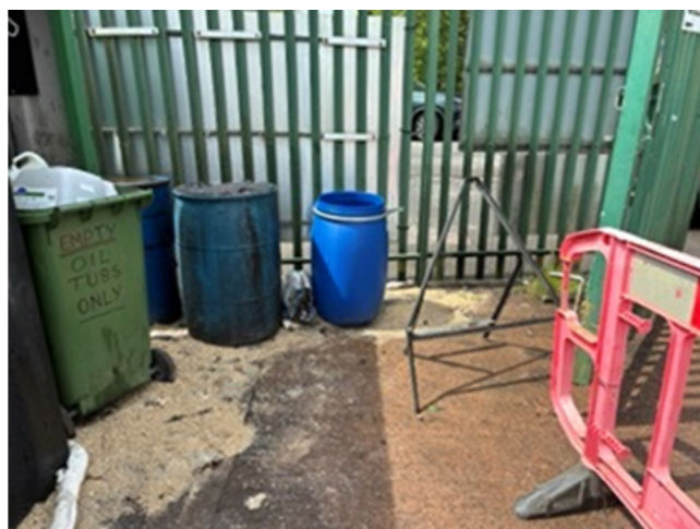
Photograph 1. Oil spill and oil drum overlapping the drainage gulley
