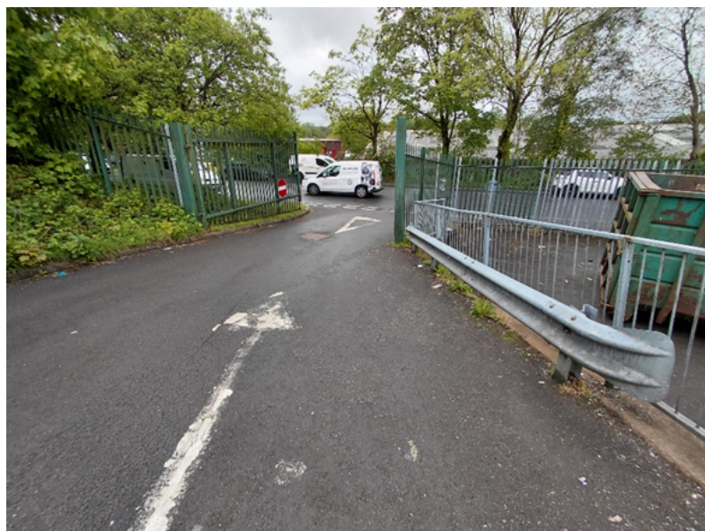
Photograph 4. Showing good housekeeping and areas of fencing that have been repaired.
