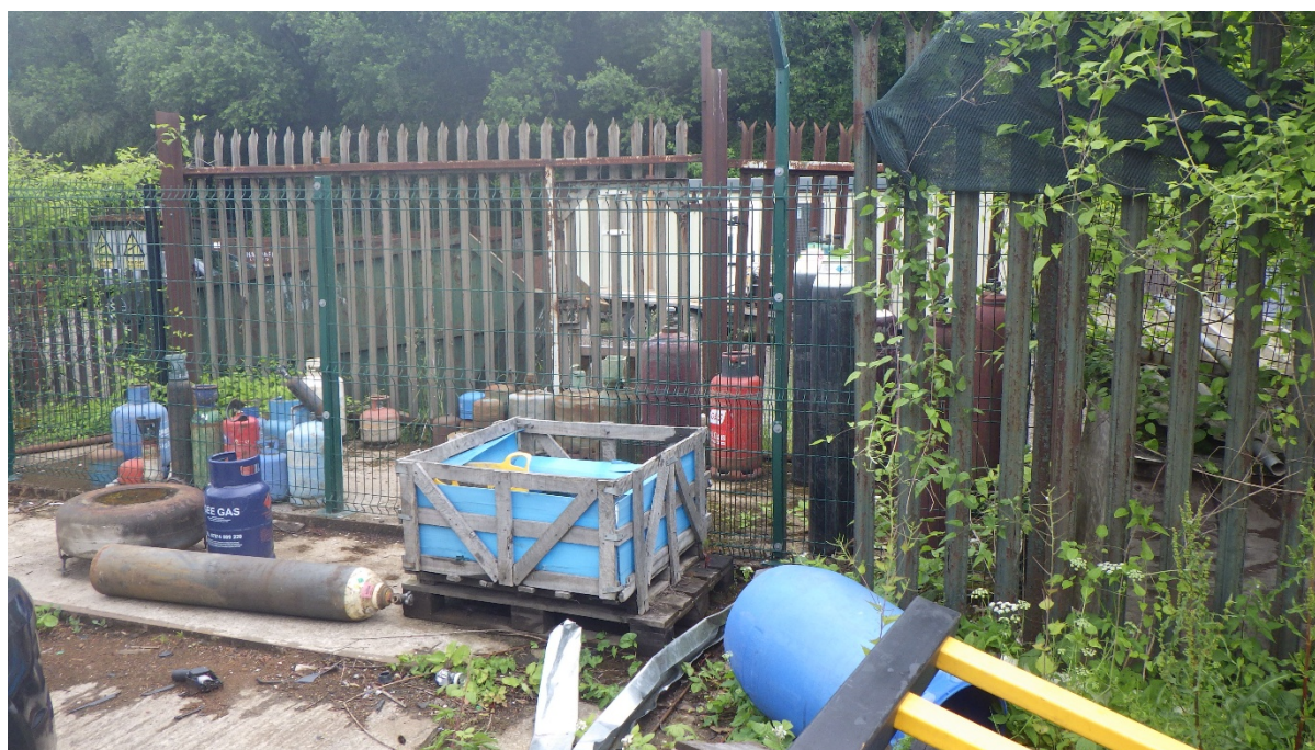
Secure storage for gas cylinders
