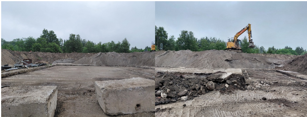
Images 3 and 4: Left – Segregation Bay awaiting renovation. Right – Segregation Bay undergoing renovation.
