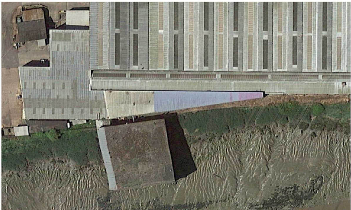
Figure 6. Aerial image of Structure B.
