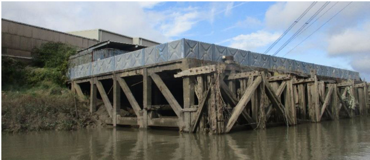
Figure 2. Photograph of the southeast corner of Structure No. 3.
