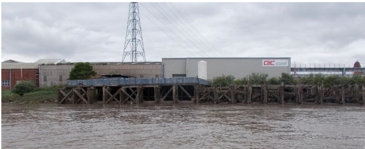
Figure 3. Photograph of front of Structure No. 3.
