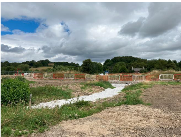
Photograph 3: Historical sluice with drainage gravel
