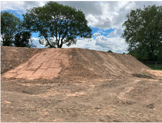
Photograph 1: Large contaminated stockpile near pedestrian entrance
