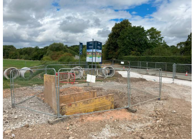
Photograph 8: Trench support in drainage area
