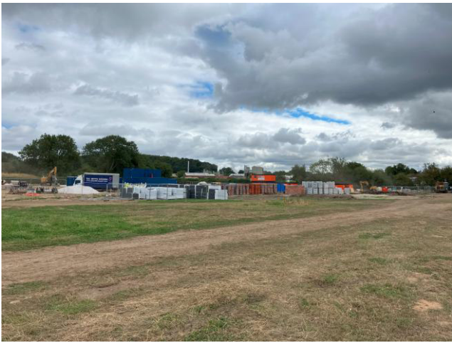
Photograph 1: Storage area in central site area
