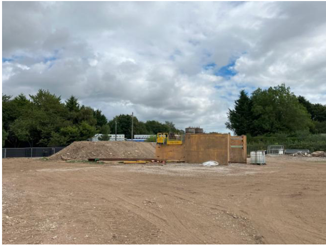
Photograph 7: Trench support and stockpile near vehicle entrance
