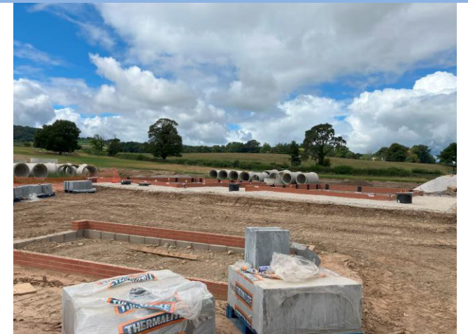
Photograph 6: Foundation bases in northern end of site
