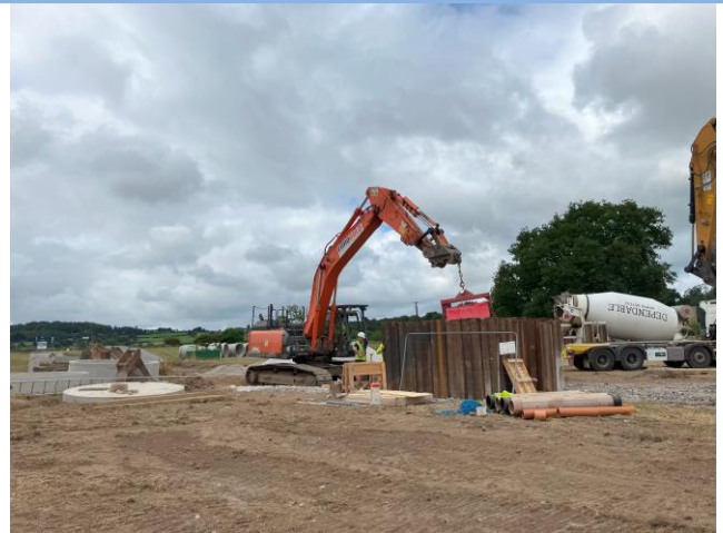
Photograph 8: Drain installation in southern road area
