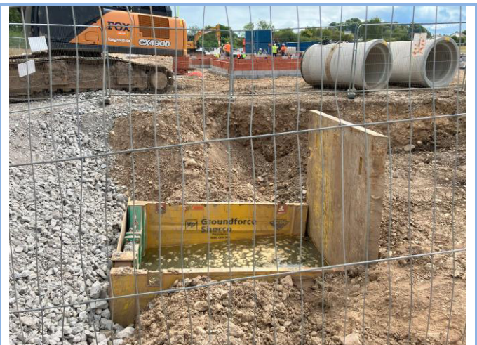
Photograph 14: Water sampling location
