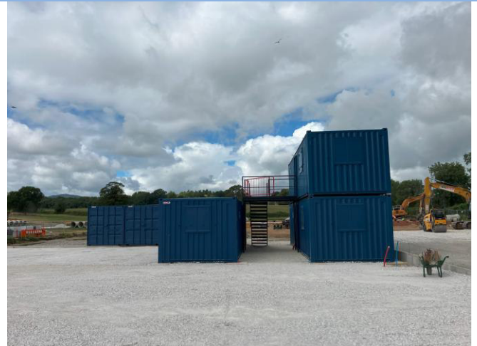
Photograph 4: New welfare and compacted MOT
