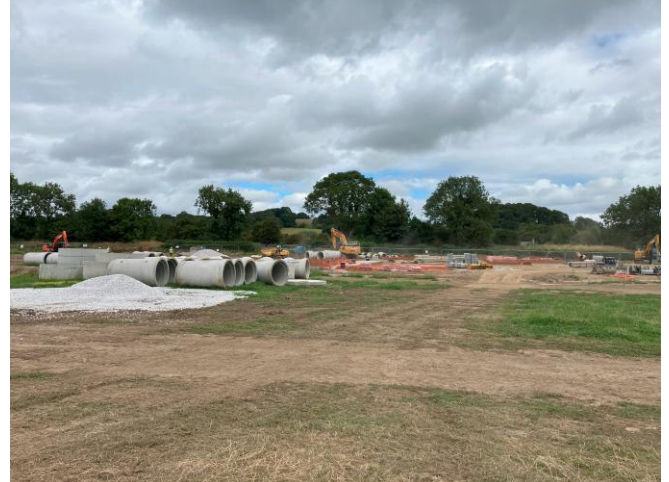
Photograph 2: Storage area in central site area
