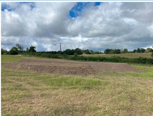
Photograph 9: TS and sod stockpiles
