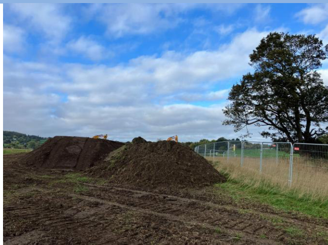
Photograph 16: Sod and topsoil stockpiles in southern central area
