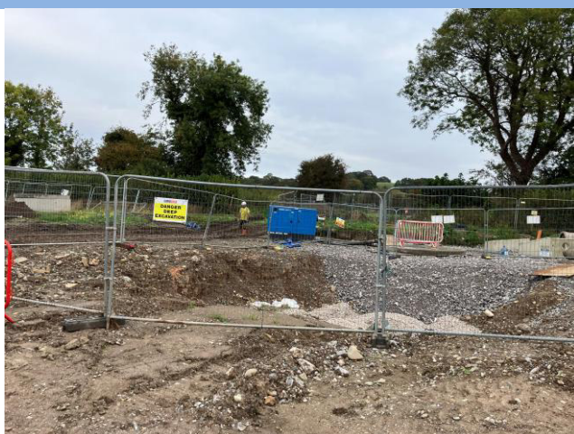
Photograph 6: Excavation with gravel fill near link road in the northwestern site area
