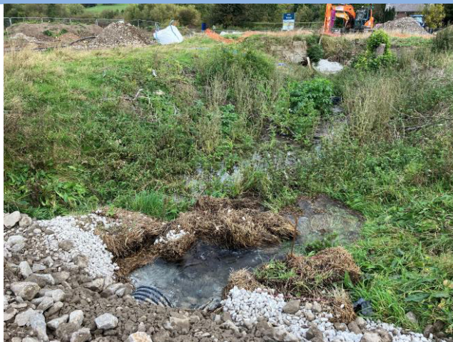
Photograph 12: Water travelling through bedding gravel and straw to historical sluice
