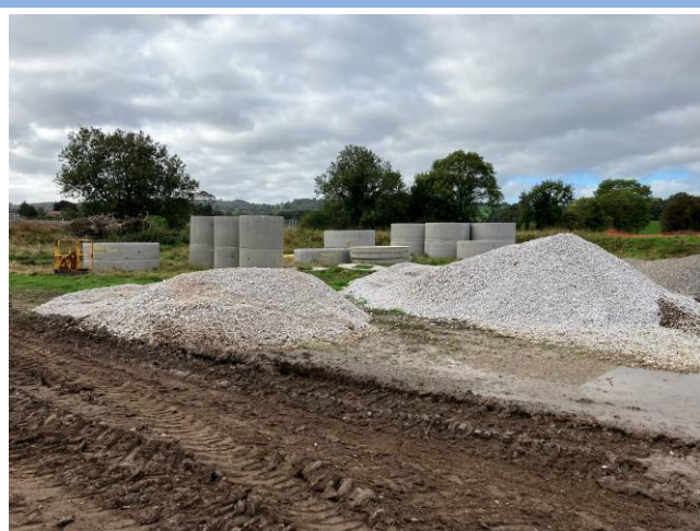
Photograph 5: Material storage area in central site
