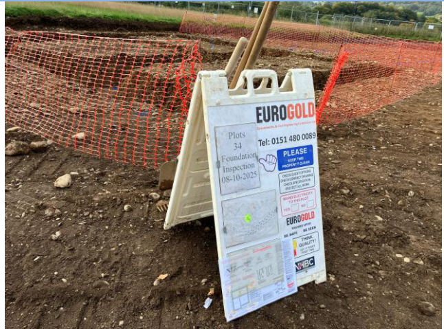
Photograph 20: Foundation inspection pit in southern site area
