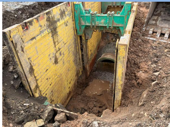
Photograph 2: Trench supports with little water
