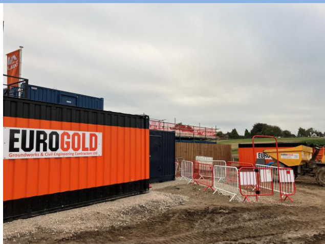
Photograph 2: New welfare area
