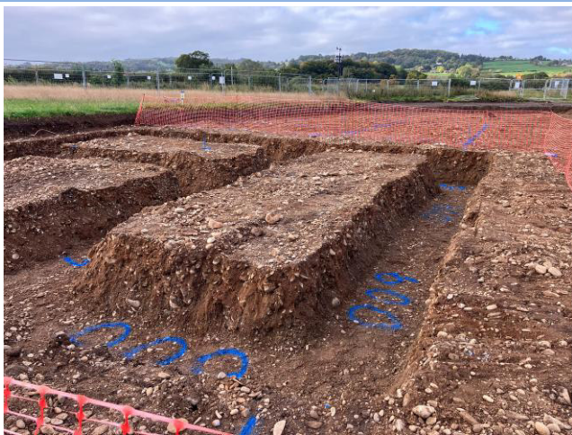
Photograph 21: Foundation inspection pit in southern site area
