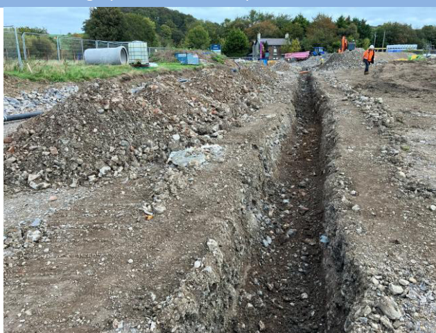
Photograph 16: Road trench in the western road area
