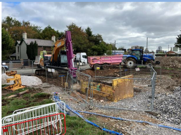
Photograph 1: Trench excavation in northeastern area
