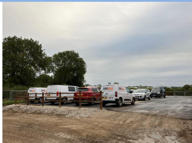
Photograph 1: Parking area next to new welfare
