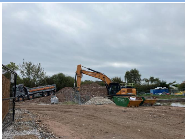
Photograph 11: Crush import in northeastern area
