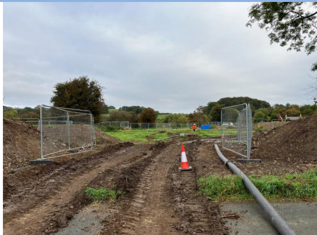
Photograph 8: Entry to northern parcel
