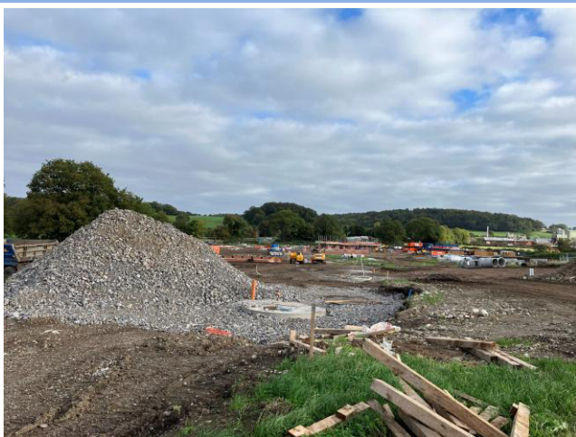
Photograph 23: Completed drain in southwestern area
