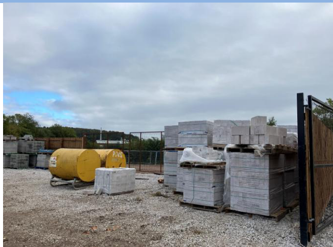
Photograph 12: Material storage next to welfare in northeastern area
