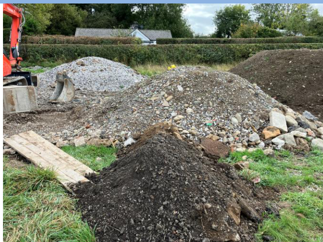
Photograph 6: Material stockpiles in eastern site area
