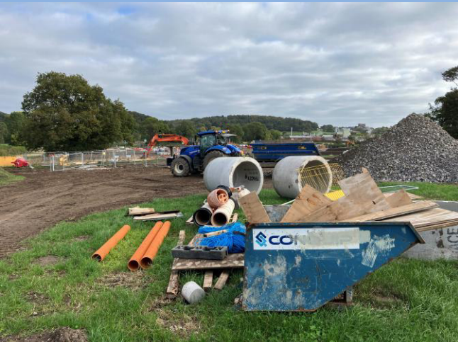
Photograph 24: Material storage in southwestern site area
