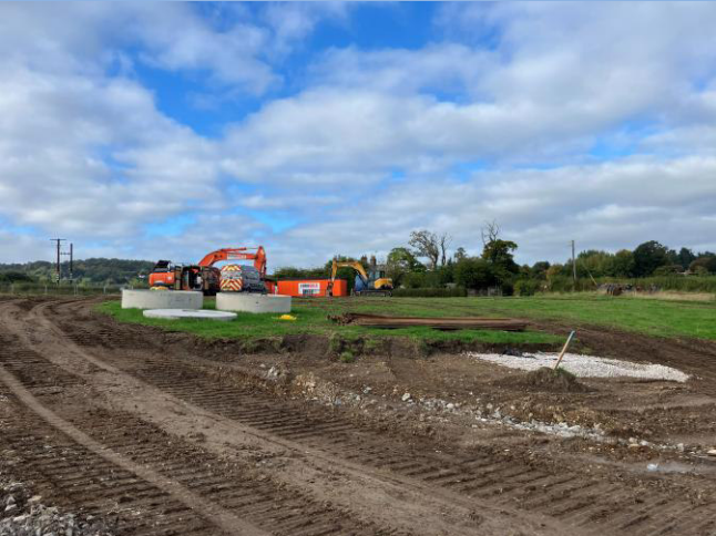
Photograph 22: Roads and sewers welfare in southwestern corner
