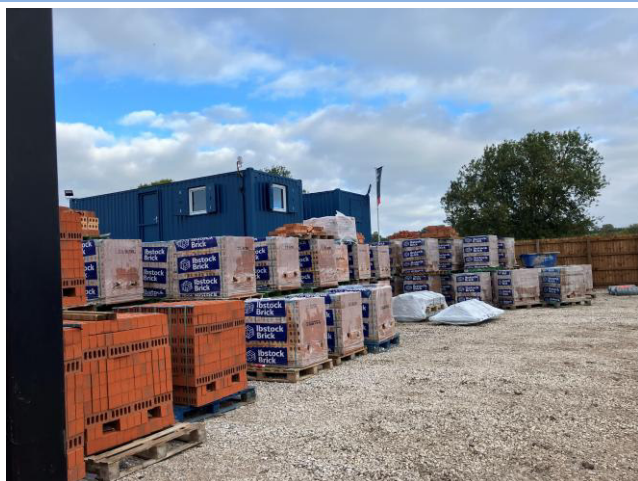
Photograph 13: Material storage next to welfare in northeastern area
