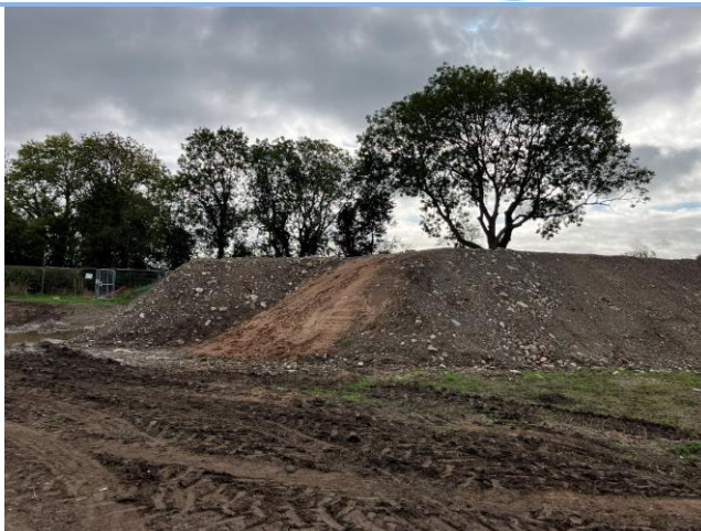
Photograph 8: Subsoil stockpile in southeastern area
