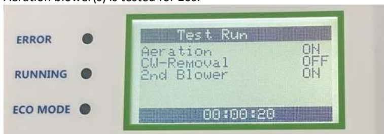
Figure 7 Aeration Blower(s) Test
