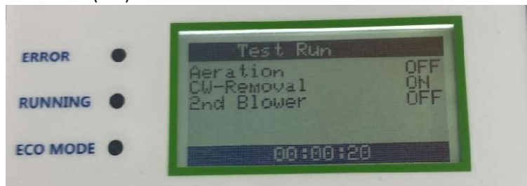
Figure 8 Clearwater Blower Test
