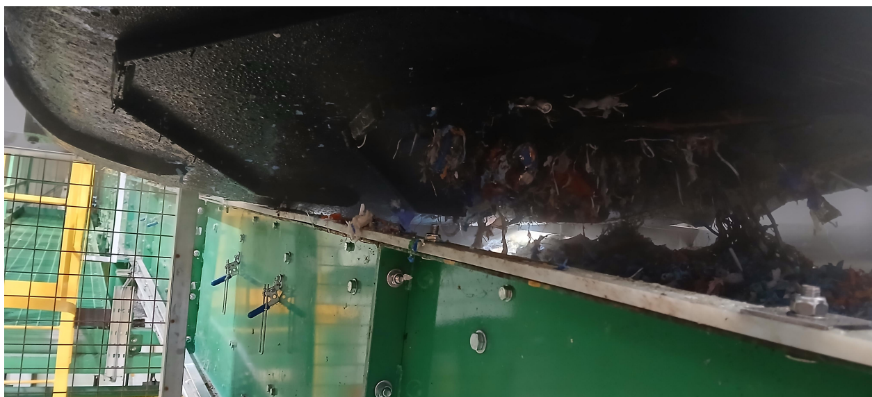
Photo 3 - Removed magnet separator which would sit on exit of line following treatment of waste(s)
