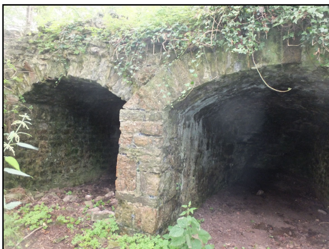
Photograph 3: Disused lime kiln building (T335) – Confirmed bat roost in 2016.
