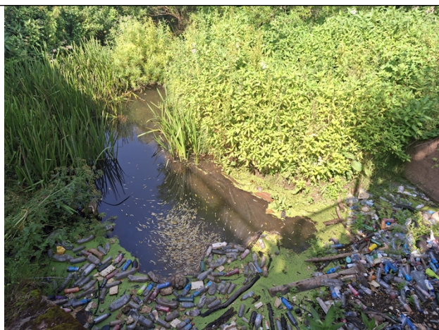
Fig 2: Upstream of impoundment structure
