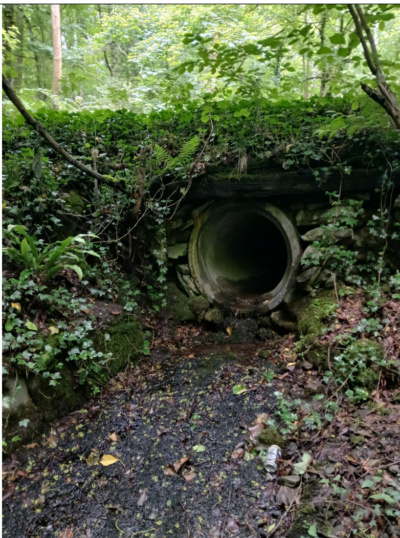
Figure 7 – 800mm pipe discharging to the leat as observed during the visit.
