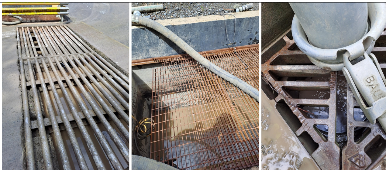
Figure 12 – The cattle grid and catchpit as observed during the visit.
