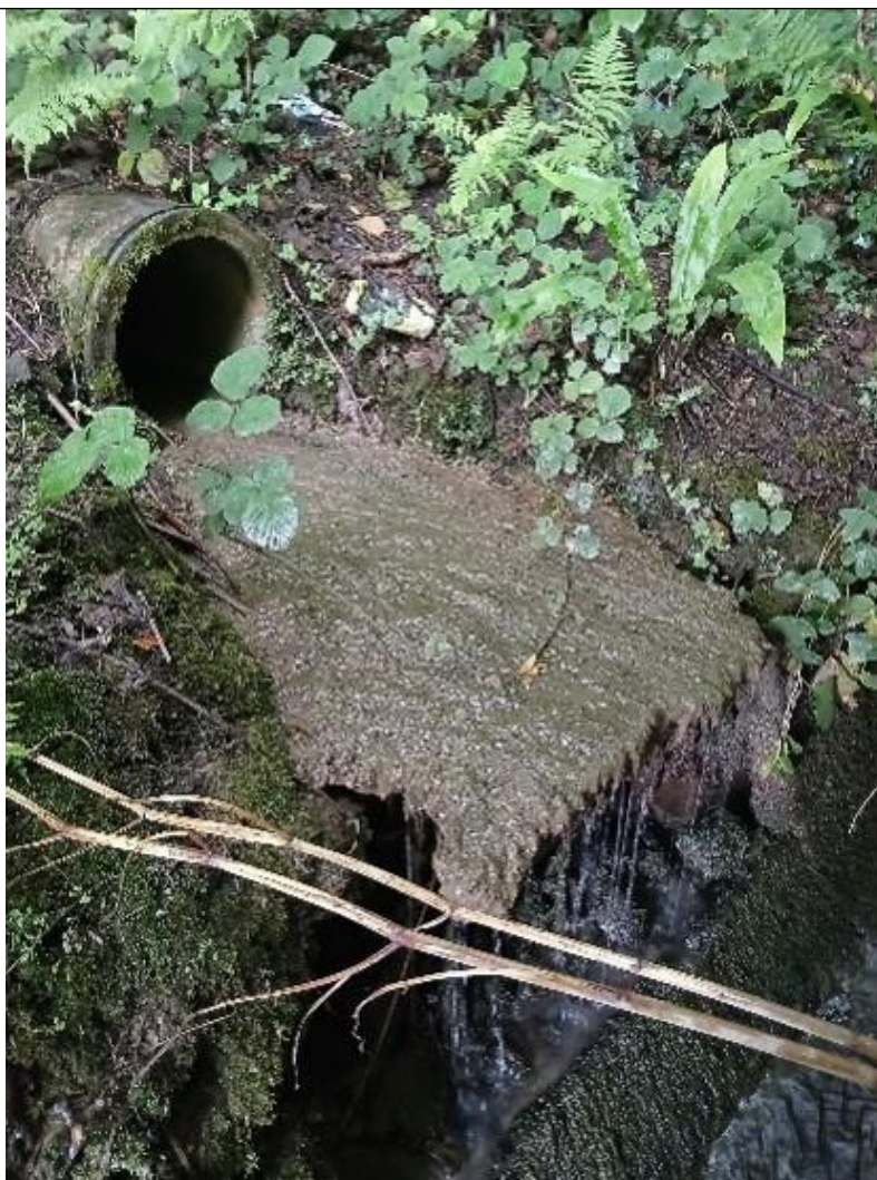
Figure 6 – Lateral pipe discharging to the leat directly upstream from the sample point.
