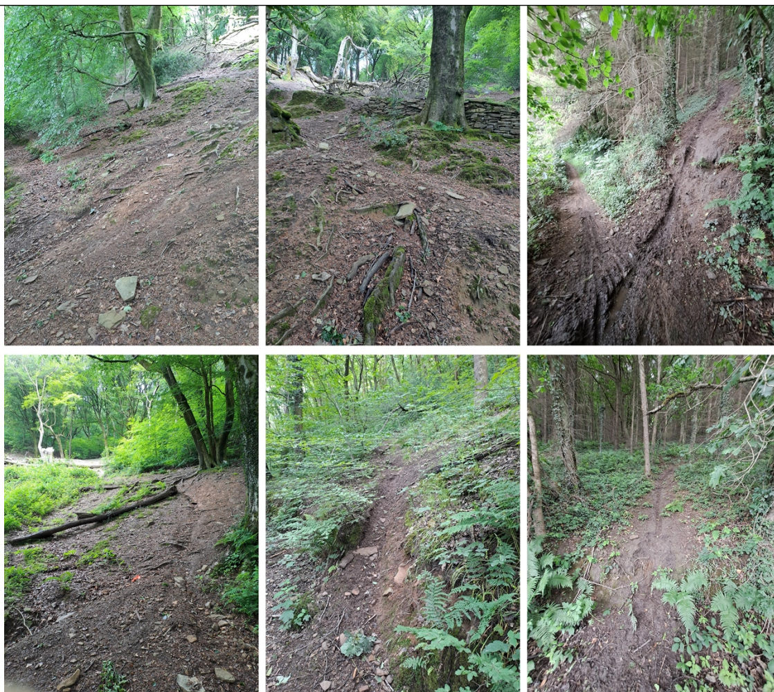
Figure 4 – An example of the areas of erosion reportedly acting as a conduit for polluted runoff.
