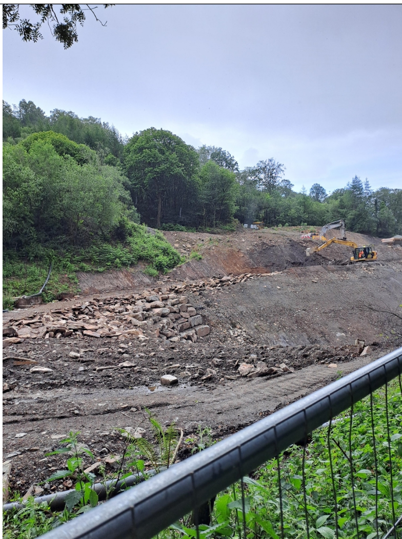
Figure 3 – Site drainage infrastructure as observed during the visit.
