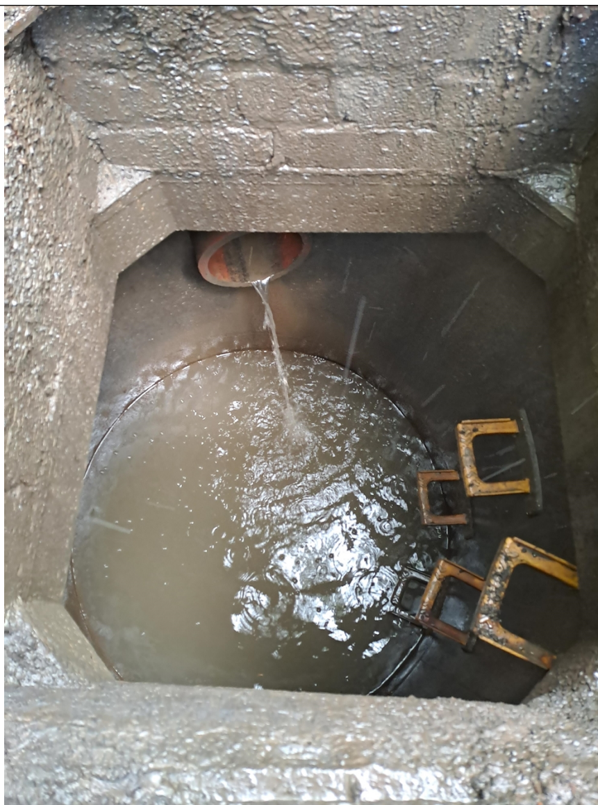
Figure 16 – The chamber identified as Silt Trap 4 as observed during the visit.
