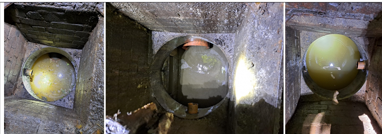
Figure 17 – Manholes 1-3 (left to right) of the drainage interceptor as observed during the visit.
