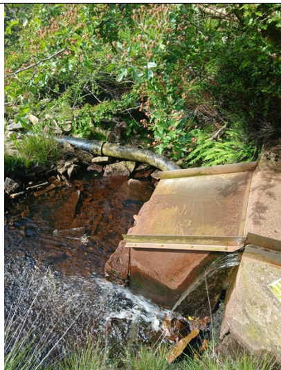
Fig 2 - Concrete Weir, Screen and Hands Off Flow Notch.
