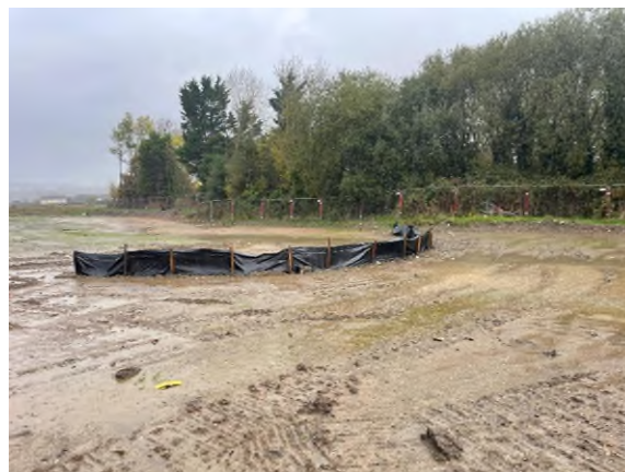
Figure 9 - Existing silt fencing installed along the north of Phase 1B
