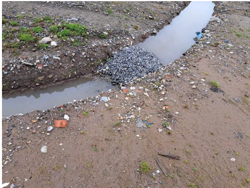
Figure 16: Example of gravel weir/bund within an open ditch
