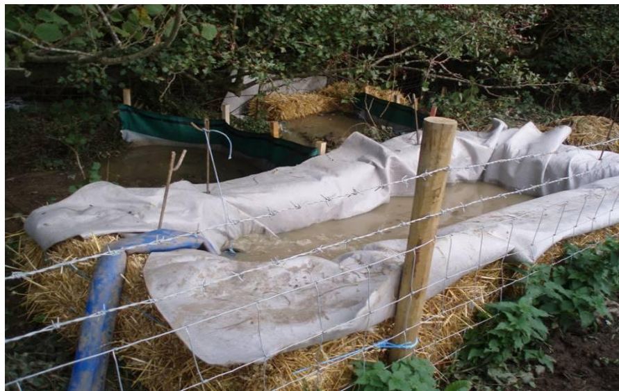
Figure 17: Bale and Geotextile Sump
