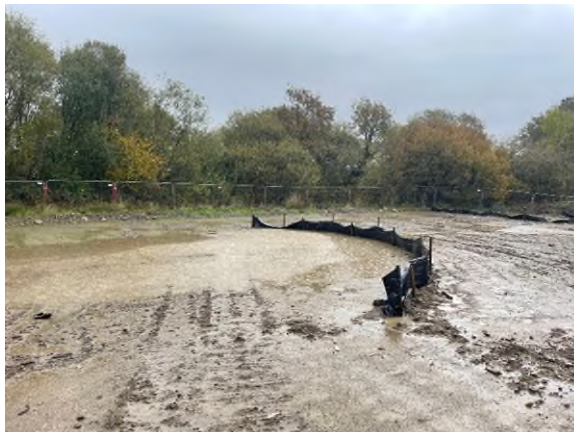
Figure 9 - Existing silt fencing installed along the north of Phase 1B
