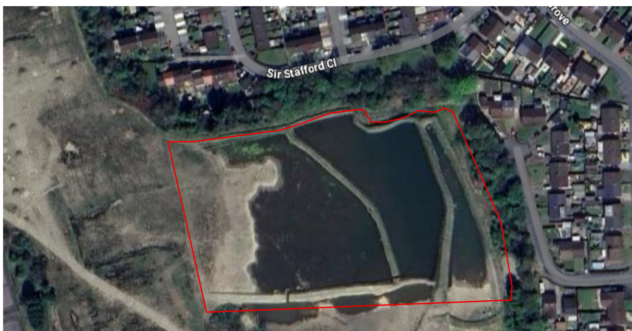
Figure 4 - Ariel image of Phase 1B, prior to remediation (ponds now removed)
