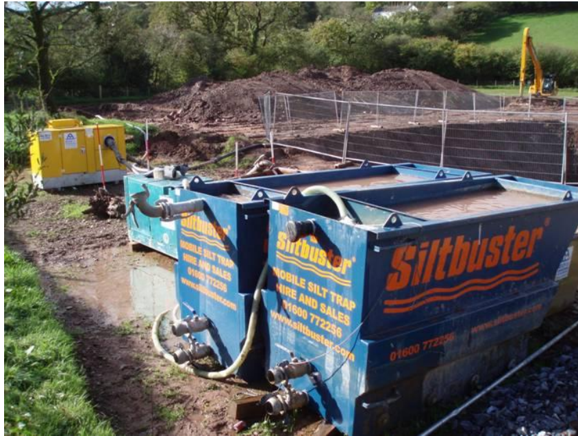
Figure 18: Pumping silt contaminated water through Lamella Clarifiers
