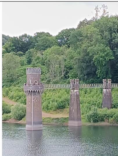
Fig 2 - Wentwood Reservoir draw off tower
