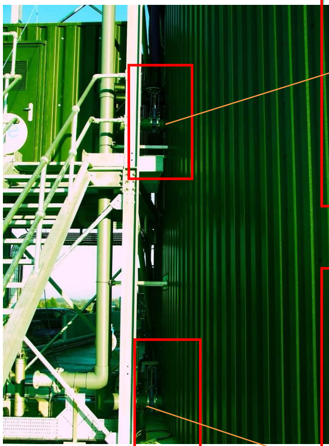
Digester Lower Unloading valves
