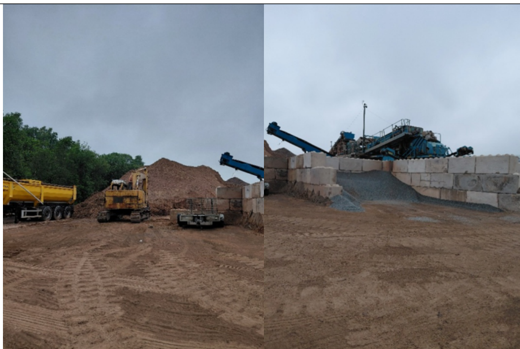
Images 2 and 3: Left – Unsorted soil/aggregate waste pile. Right – Treated soil/aggregate waste material in a segregated bay.
