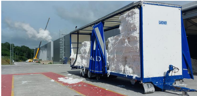
Photograph 1-1: HGV unloading area
