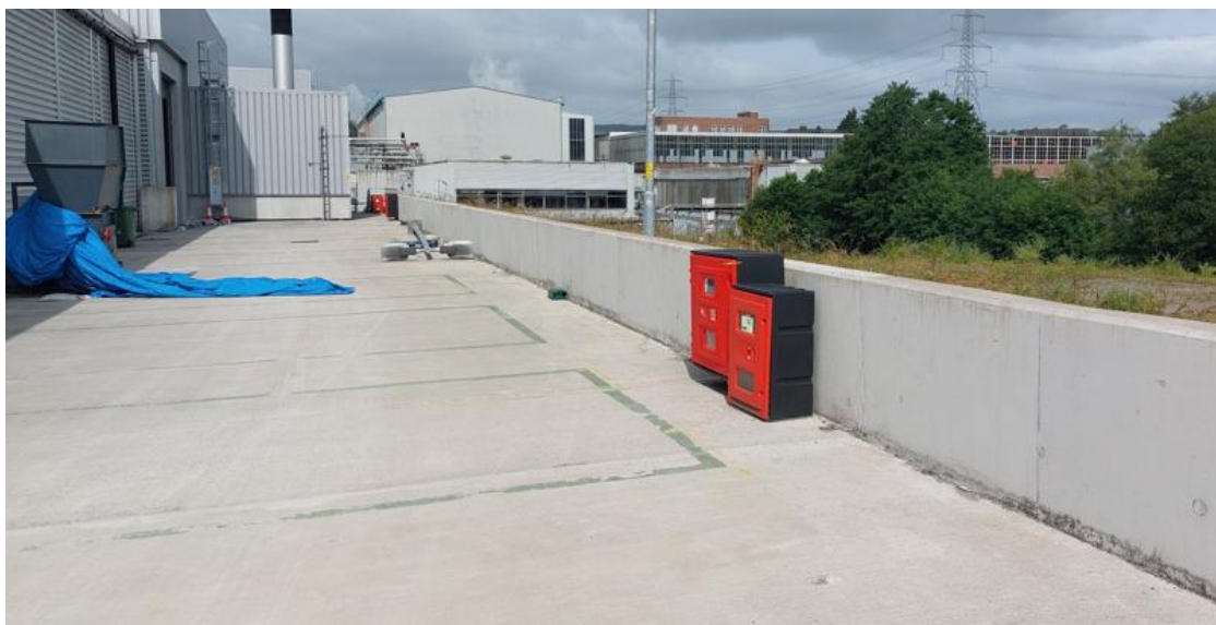
Photograph 9-2: Department A retaining wall
