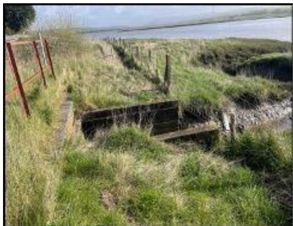
Figure 8: Vegetation surrounding culvert (East side).
