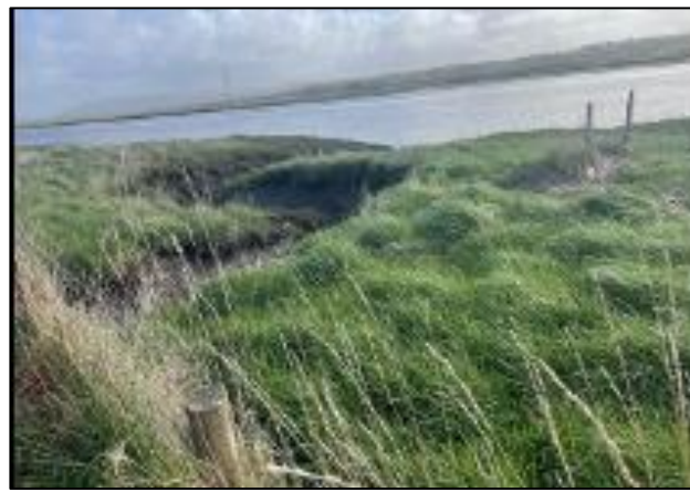
Figure 9: Vegetation surrounding culvert (West side).
