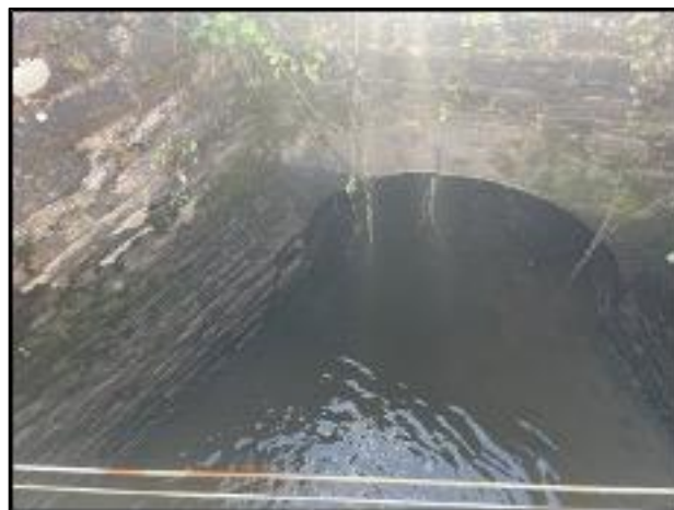
Figure 5: Watercourse beneath culvert.
