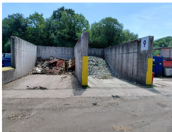
Image 4: External segregation bays in the waste transfer station area for wood and glass.
