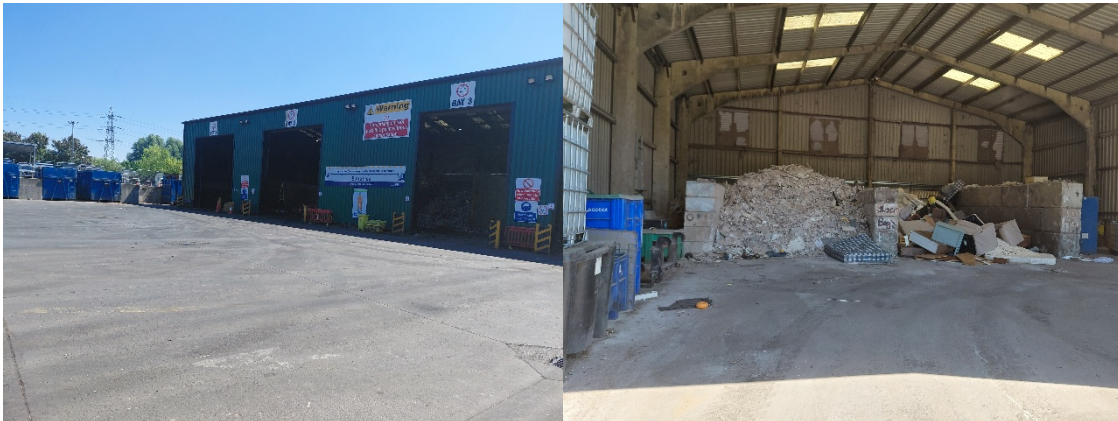
Images 4 and 5: Left – waste transfer station for recyclables and general waste. Right – internal storage of plasterboard and furniture.
