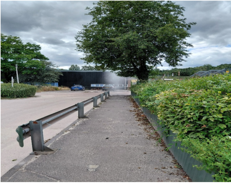
Photo 1 – Showing water sprinkler on entrance to site
