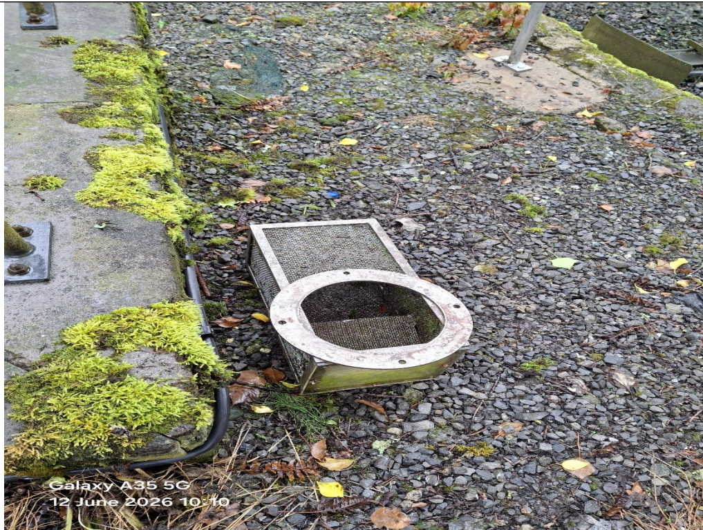
Figure 1 Storm screen not currently in position as it blinds and clogs during storms. END.
