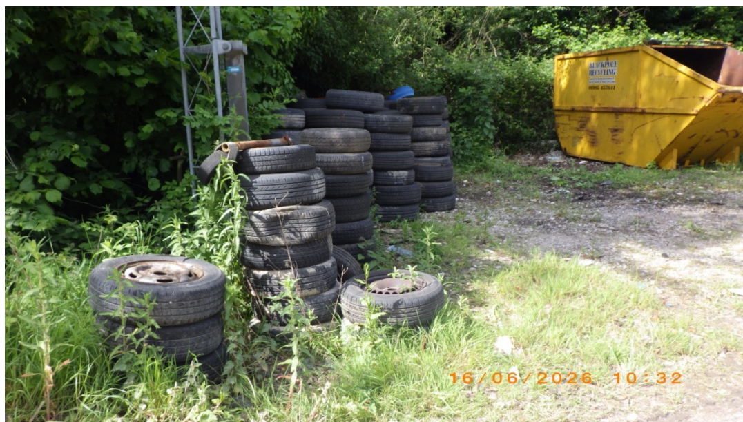
Tyres stored next to a skip marked on the site plan as the storage of tyres in a 8yard skip
