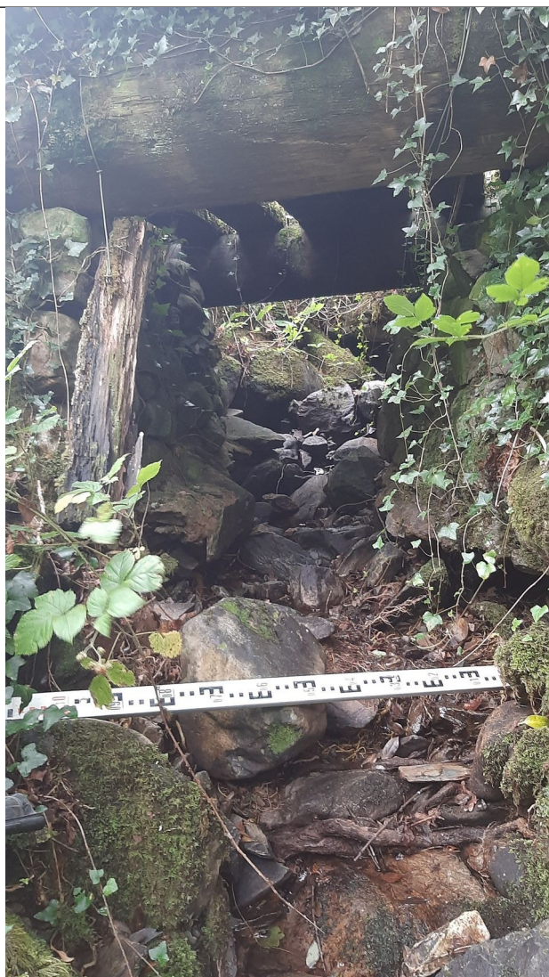
Figure 17 - View beneath bridge showing stone abutments
