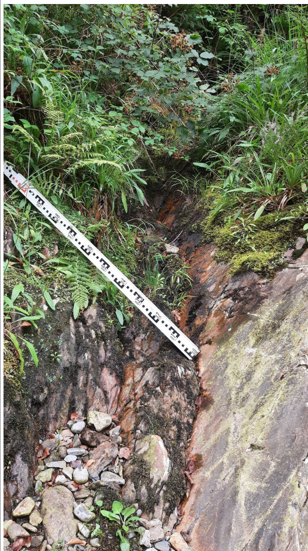
Figure 6: Downstream end of tailrace
