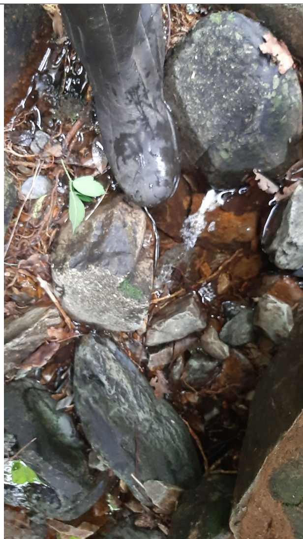
Figure 18 -Bed substrate beneath bridge
