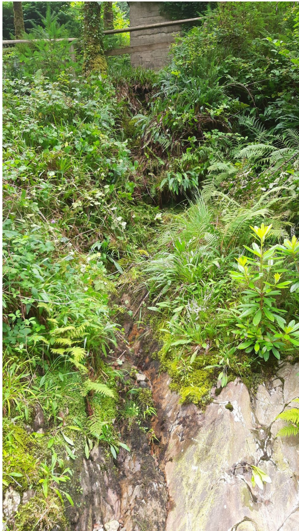
Figure 7: Tailrace viewed from downstream
