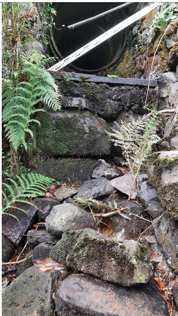
Figure 23 – downstream end of culvert
