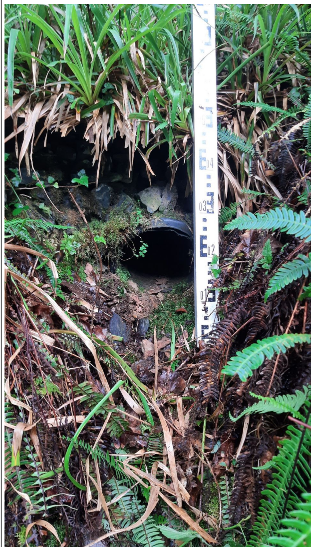
Figure 5: Outfall pipe
