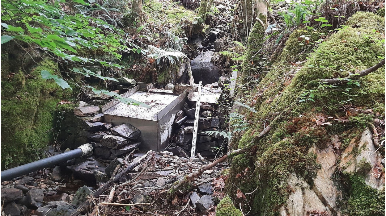
Figure 1: View from downstream 1
