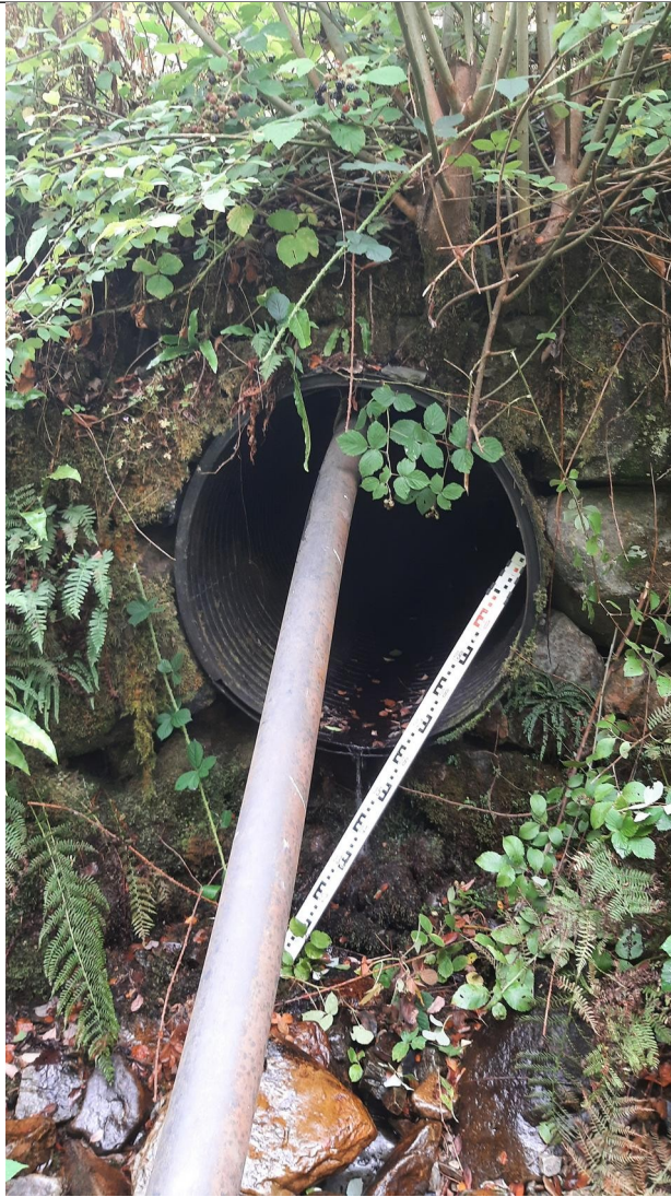
Figure 21 - Downstream end of culvert
