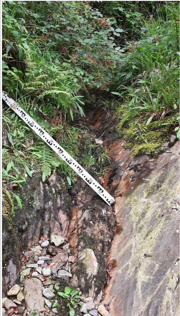
Figure 6: Downstream end of tailrace
