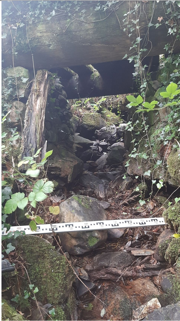
Figure 17 - View beneath bridge showing stone abutments
