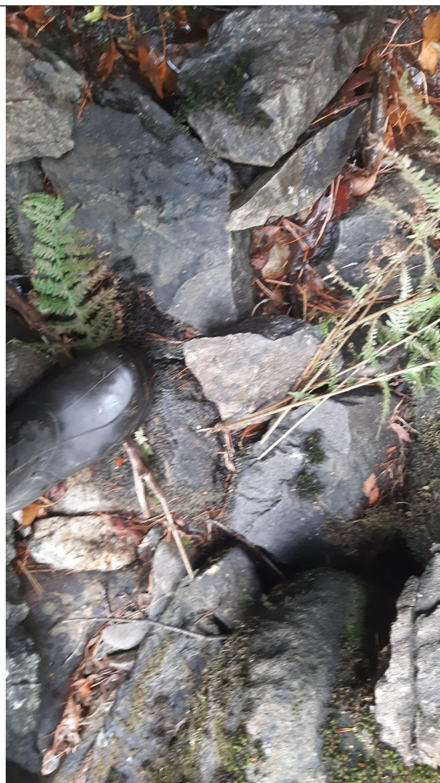
Figure 24 – Bed substrate downstream of culvert
