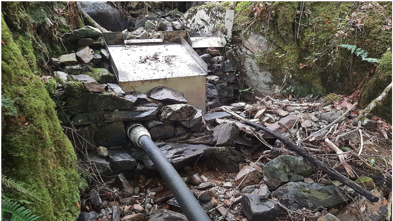
Figure 2: View from downstream 2
