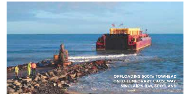
1 OF 2 COMPRESSORS, BELLISWICK BAY, PEMBROKE
