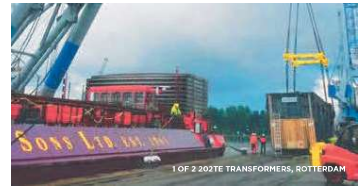
1 OF 2 202TE TRANSFORMERS, ROTTERDAM
