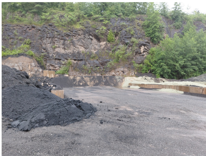
Figure 3: Segregated bays for waste types
