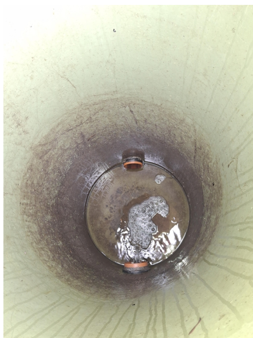
Fig1: Inspection chamber of system 1
