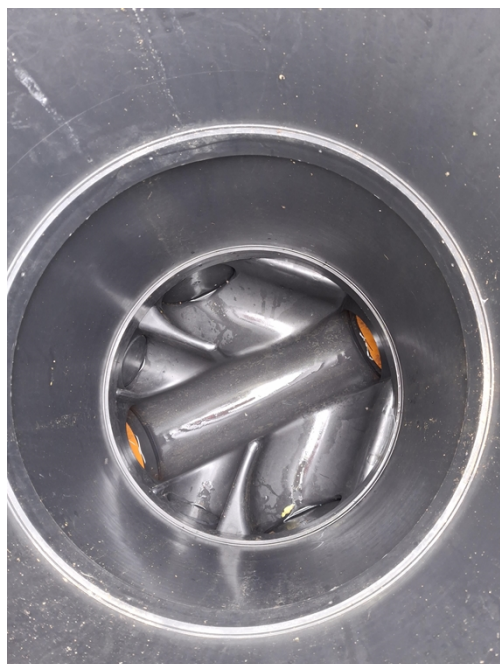
Fig2: Inspection chamber of system 2
