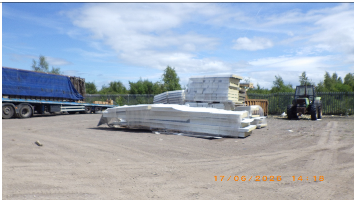
Panels stored at the back of the site
