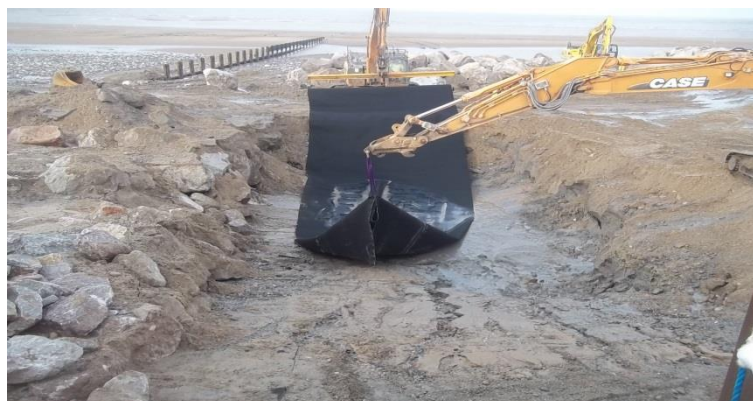
Figure 18- Typical geotextile placement
