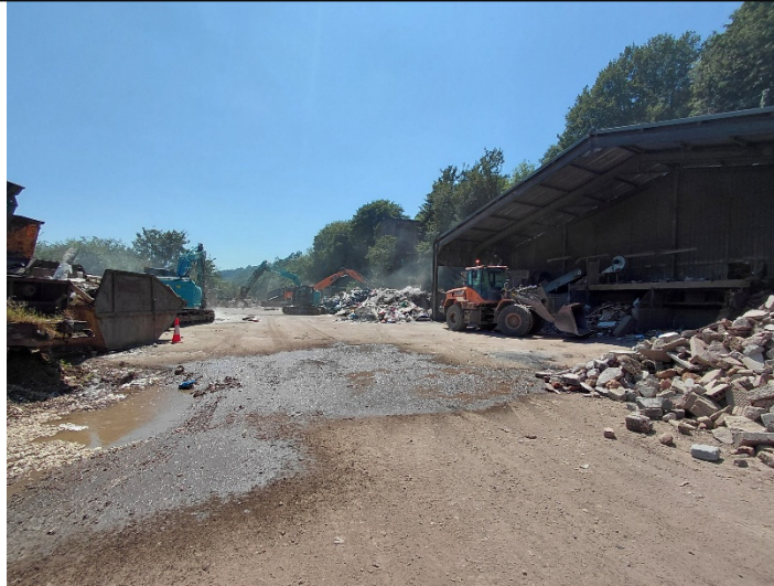
Image 1: Sprinklers in operation on the top yard.
