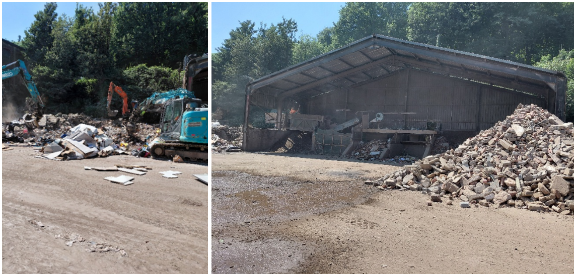
Images 2 and 3: Left – Unsorted waste pile undergoing waste operations. Right – Weatherproof segregation bays for aggregate type materials.
